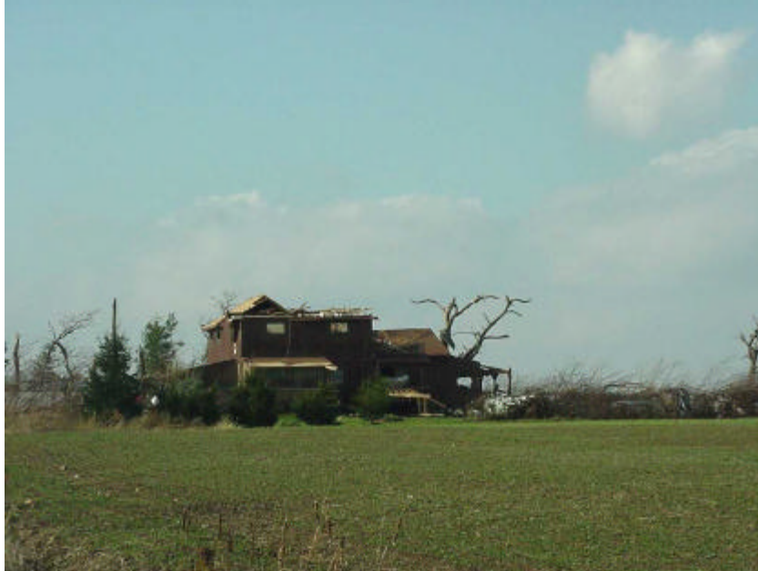
Wayne County tornado damage along Easton Road near West Salem.
