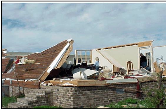
Above: An F2 tornado, as defined by the Fujita Tornado Scale with wind speeds between 113 and 157 mph hit the Bedford County community of Bugscuffle at 1745 (5:45 pm) CST. Several houses were damaged and destroyed. (Photo courtesy: Ralph Troutman, DAPM, NWS Nashville, Tennessee.)
