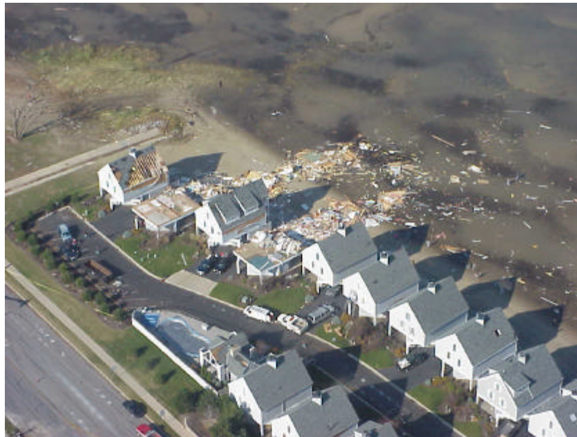
Port Clinton tornado damage along Lake Erie near Lakeview Park.
