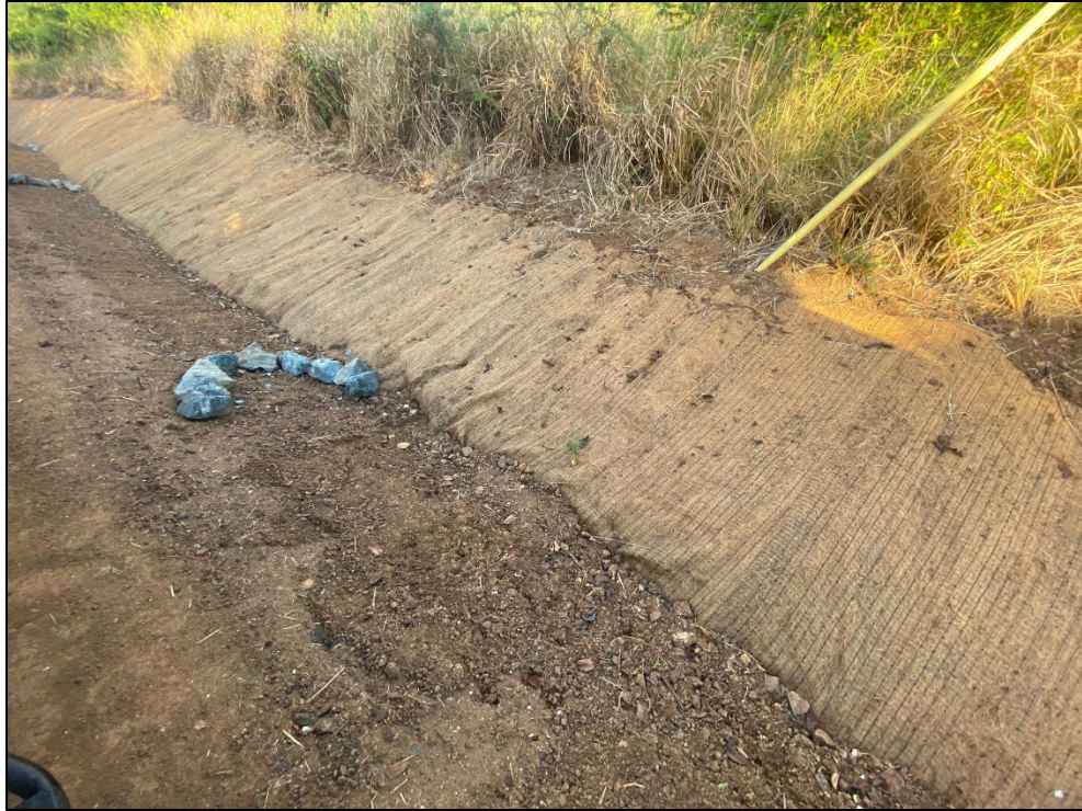
Figure 13 Stabilized cutslope with erosion control mat.
