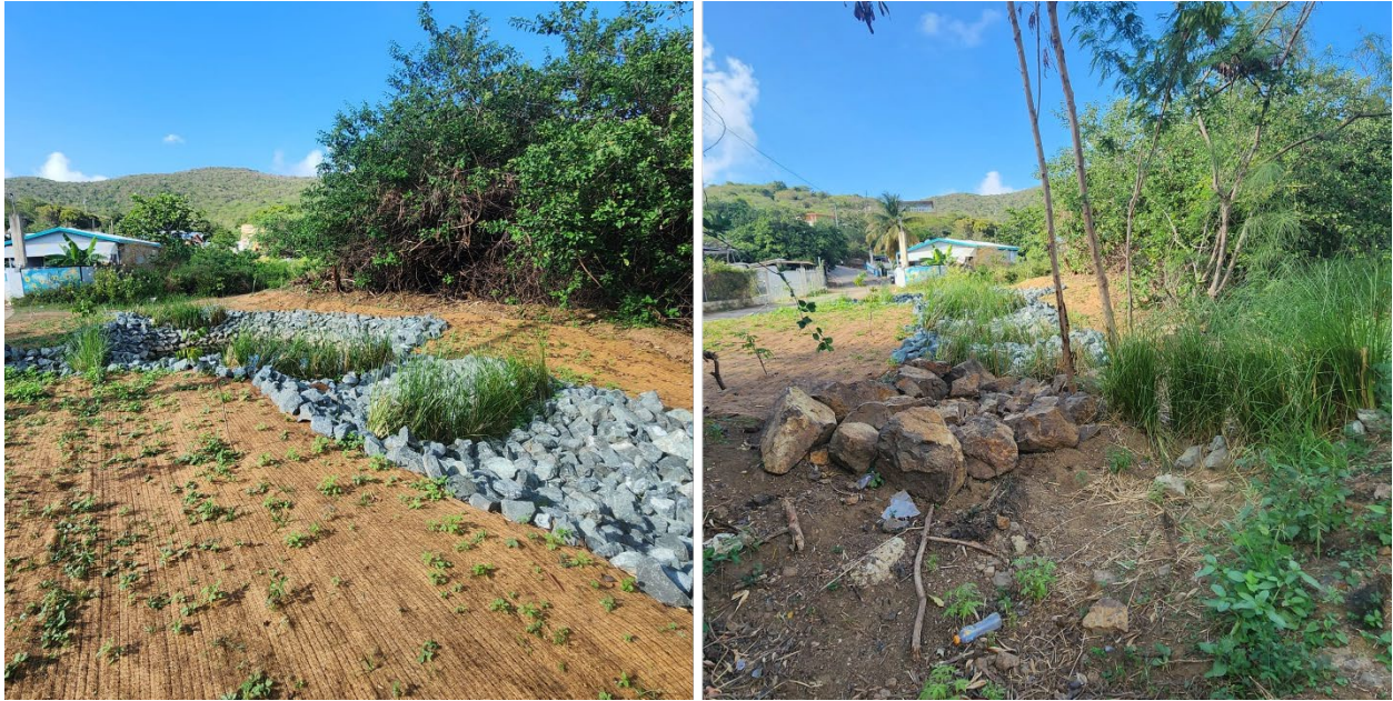
Figure 20 Sediment trap and stabilized outlet and swale constructed at Coronel watershed road segment CO-21B.
