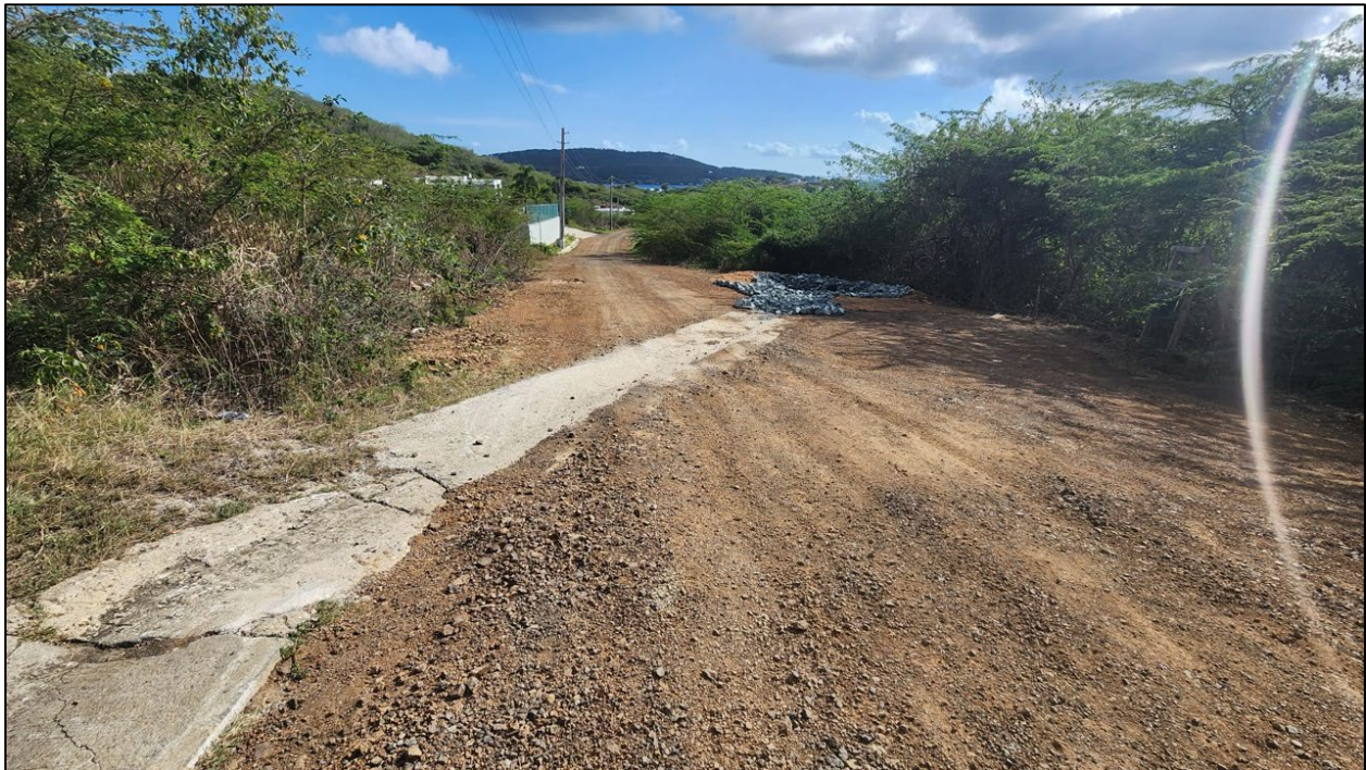
Figure 17 Sediment Traps and swales constructed in Coronel watershed in Segment CO-21B.
