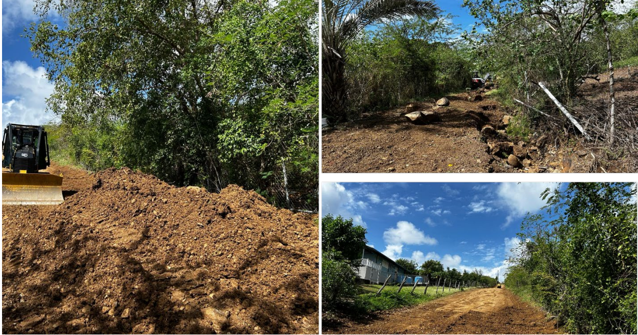
Figure 9 Grading, compacting and ditch construction at Coronel watershed, road segment CO-21B.
