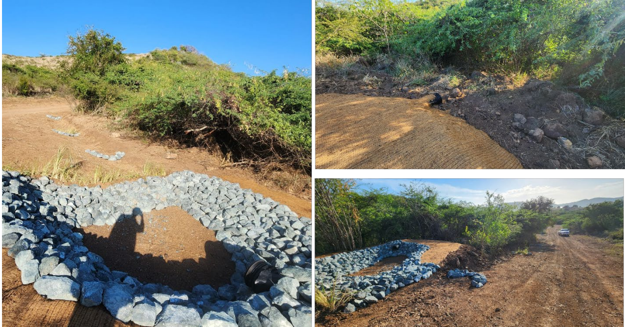
Figure 18 Sediment Trap installed at Carenero watershed in road segment Carenero-2.
