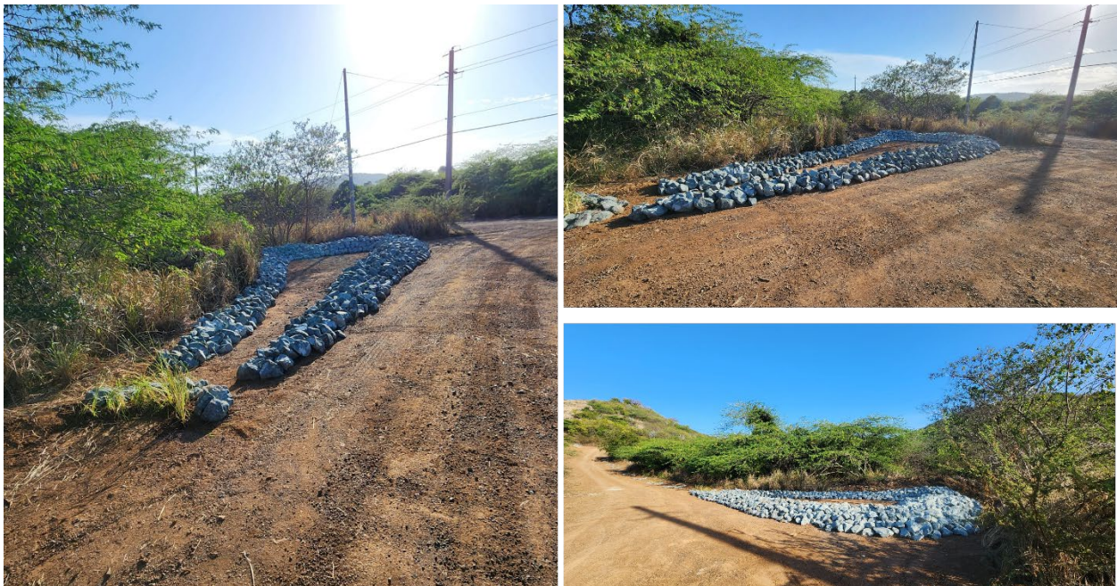
Figure 19 Sediment Trap designed to receive runoff from ditch with check dams at Carenero-2 road segment.
