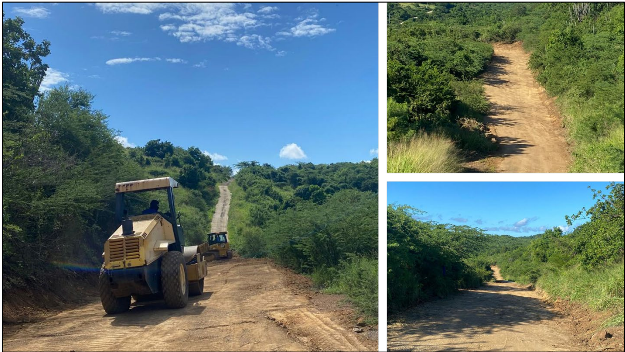
Figure 8 Grading and compaction of road prior to implementation of BMPs.
