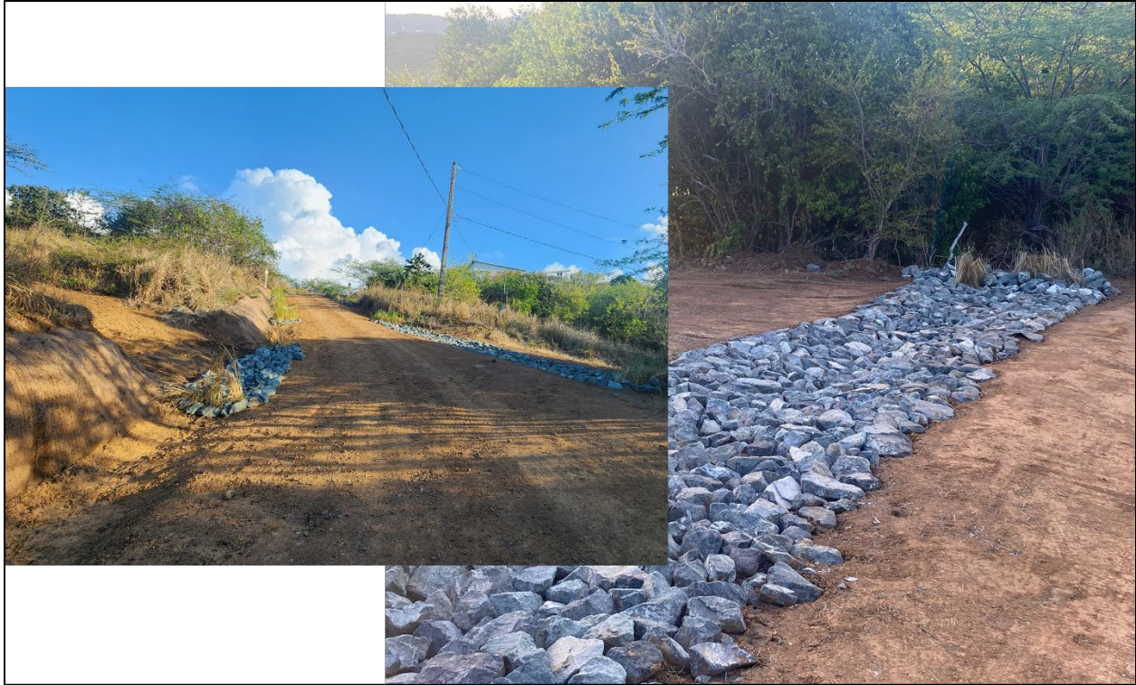
Figure 14 Swale redirecting runoff to forested area at Cabra Watershed (Segment CA-11).
