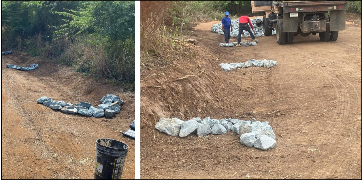
Figure 12 Check Dams and sediment detention pond being constructed in road segment Carenero-2.
