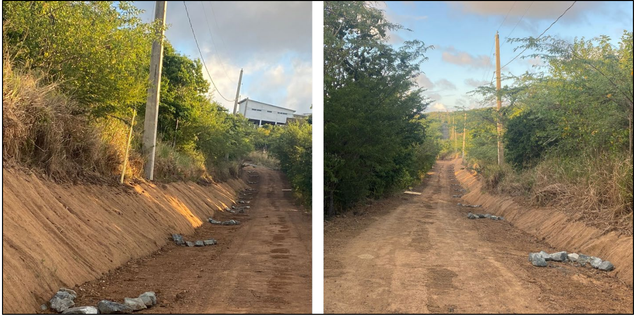
Figure 10 Stabilized road segment (CA-11) in Cabra Watershed. The road was insloped to a ditch and check dams were located in the ditch. The cutslope was protected with an erosion control mat. Left picture: Looking upslope. Right picture looking downslope.
