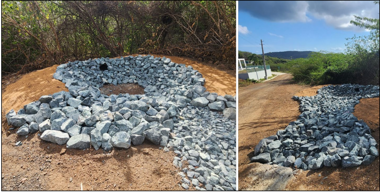
Figure 16 Sediment Traps and swales constructed in Coronel watershed in Segment CO-21B.
