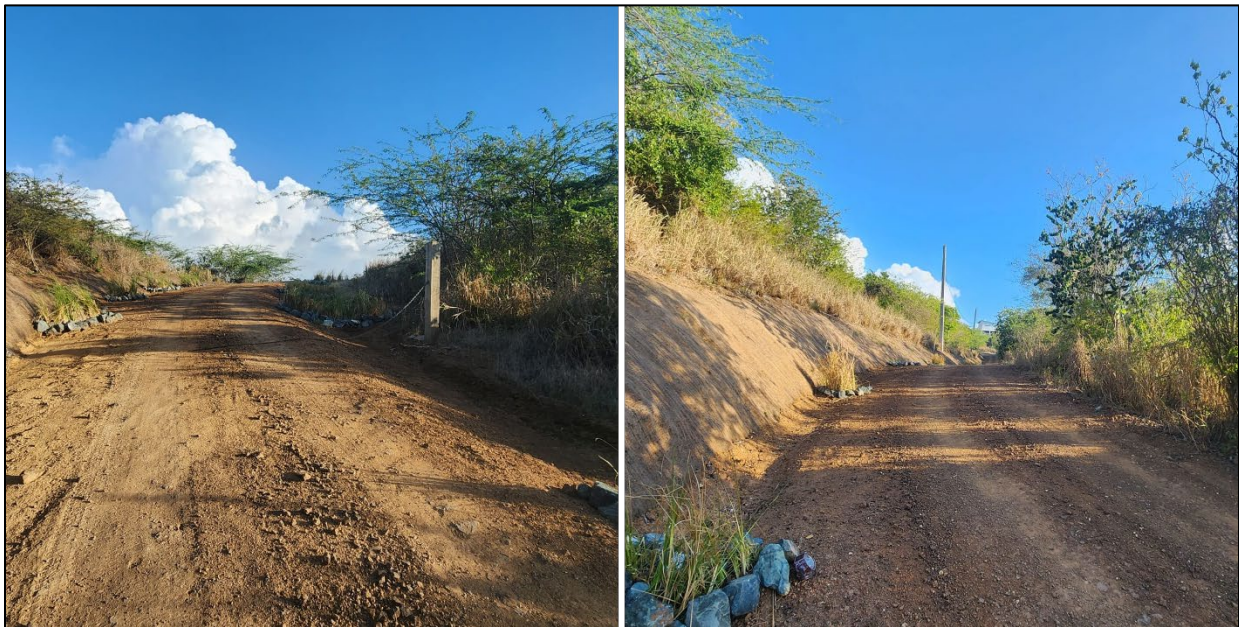
Figure 11 Check dams finalized and with planted vetiver at road segment CA-11 in Cabra watershed. Note the cutslope stabilized with an erosion control mat.
