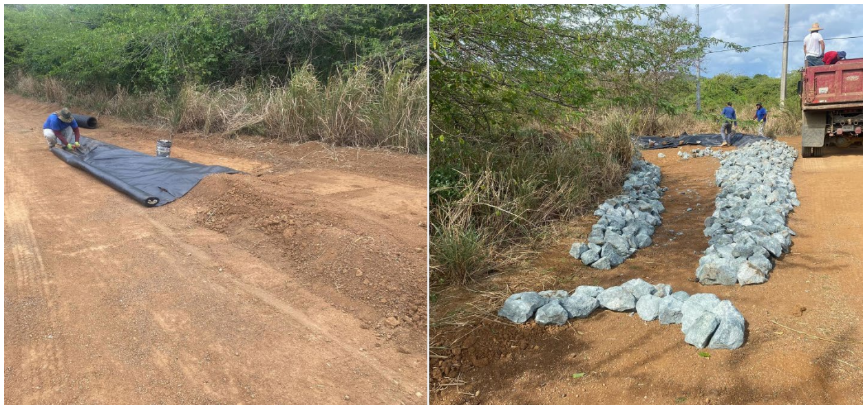
Figure 15 Installation of geotextile and berm to construct inlet to sediment trap at Carenero watershed in road segment Carenero-2.
