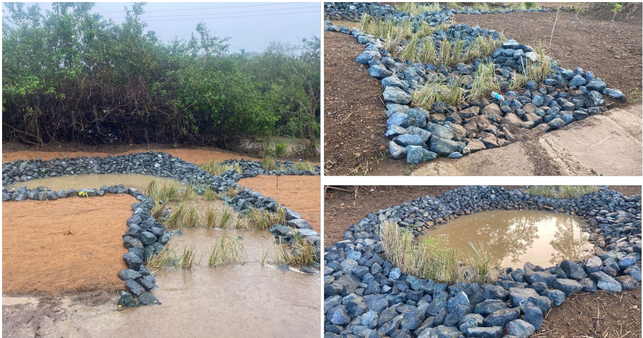
Figure 21 Evidence of sediment traps at Coronel watershed (CO-21B) receiving runoff and sediment.
