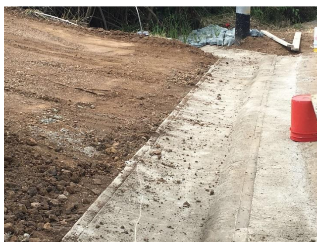
Figure 45. Example of swales made by PDC in Culebra (concrete) and in a coffee farm (stones).
