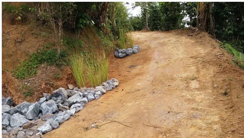
Figure 40. Example of check dams constructed by PDC on a dirt road network in coffee farms of Yauco Puerto Rico.
