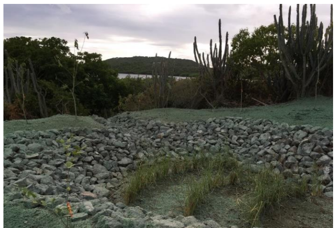
Figure 27. BMP's implemented following a train treatment approach in Puerto del Manglar in Culebra, Puerto Rico. Practices include bioswales and sediment traps.
