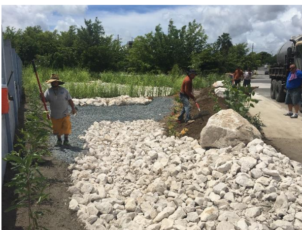
Figure 28. BMP's implemented following a train treatment approach in Yauco, Puerto Rico. Practices include bioswales, bioretentions and raingardens.
