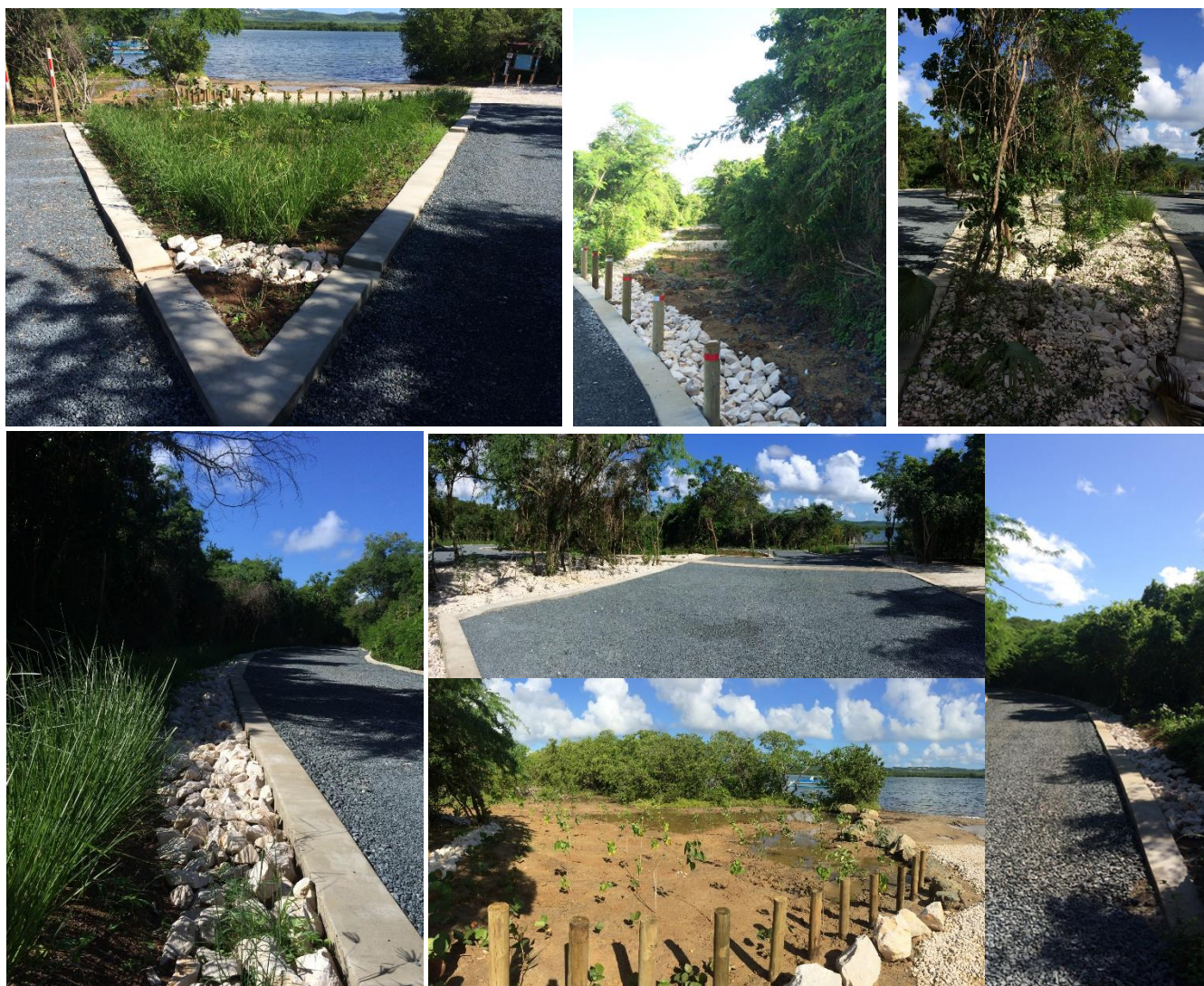
Figure 23. BMP's implemented following a train treatment approach in Mosquito Bay in Vieques Puerto Rico. Practices include bioswale, bioretention, raingardens, constructed treatment wetlands and permeable parking.
