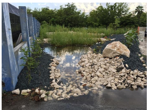
Figure 28. BMP's implemented following a train treatment approach in Yauco, Puerto Rico. Practices include bioswales, bioretentions and raingardens.
