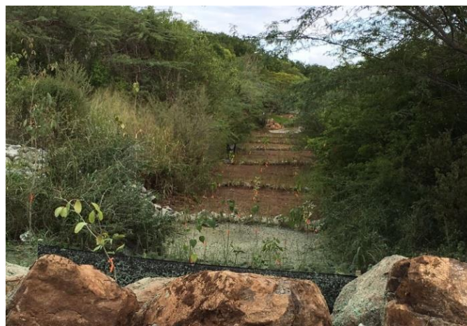
Figure 27. BMP's implemented following a train treatment approach in Puerto del Manglar in Culebra, Puerto Rico. Practices include bioswales and sediment traps.
