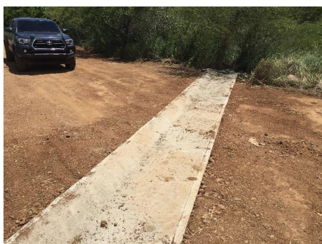
Figure 45. Example of swales made by PDC in Culebra (concrete) and in a coffee farm (stones).
