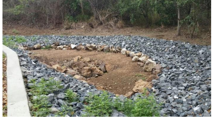
Figure 25. BMP's implemented following a train treatment approach in Punta Soldado in Culebra, Puerto Rico. Practices include bioswales, bioretentions, raingardens, sediment traps and permeable parking.
