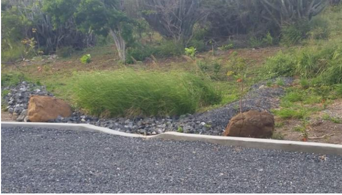
Figure 25. BMP's implemented following a train treatment approach in Punta Soldado in Culebra, Puerto Rico. Practices include bioswales, bioretentions, raingardens, sediment traps and permeable parking.
