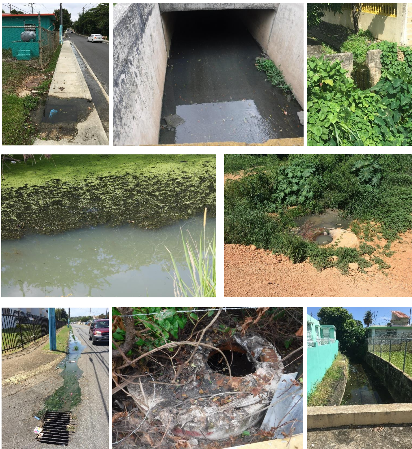
Figure 8. Examples of failing sewer infrastructure across the RFW area. Images provided by Hector Sanchez from the Fajardo Municipality Planning Board and PDC staff. Pictures are from 2014, 2016 and 2017 showing persistent problems of sewage overflows.
