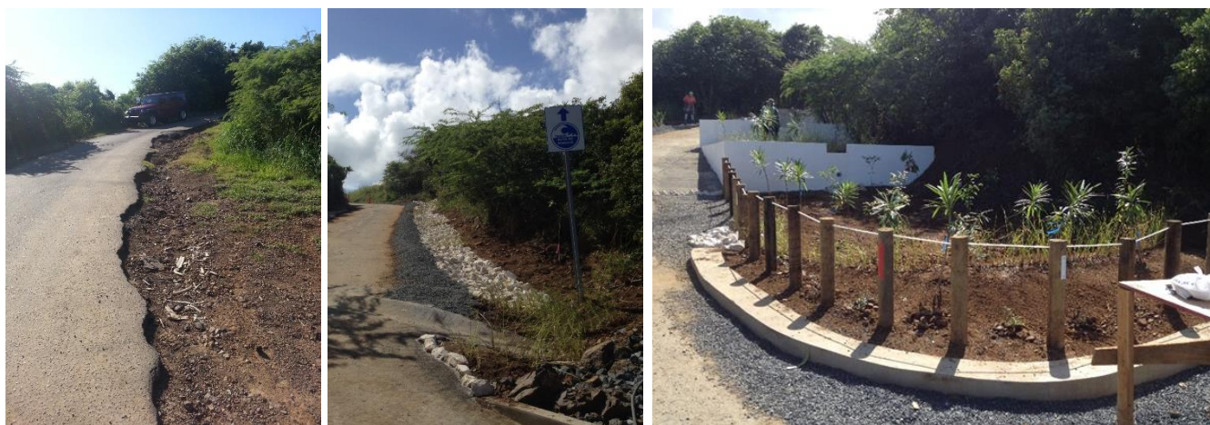
Figure 24. BMP's implemented following a train treatment approach in Zoní Beach at Culebra Puerto Rico. Practices include bioswales, bioretentions, raingardens and permeable parking.
