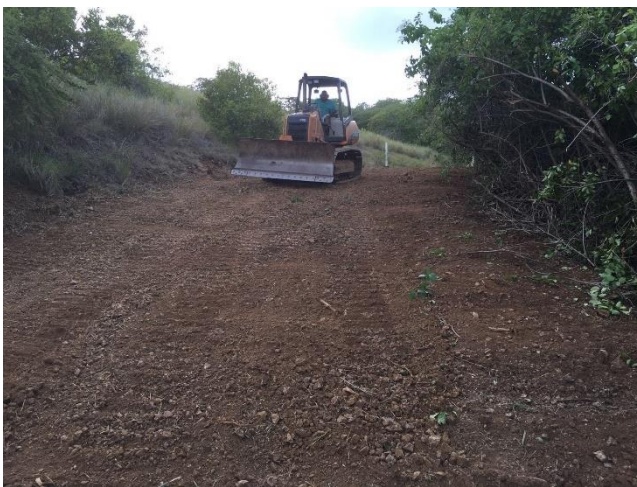
Figure 39. Example of regrading and compaction by PDC on a dirt road in Culebra, Puerto Rico.
