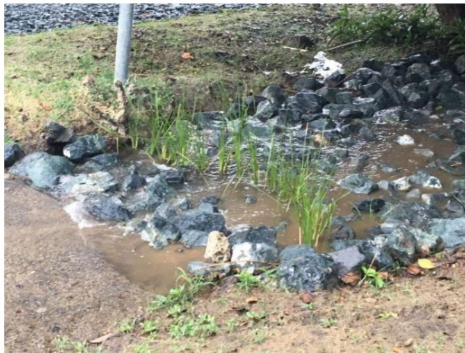
Figure 26. BMP's implemented following a train treatment approach in Fulladosa Culebra, Puerto Rico. Practices include bioswales and raingardens.
