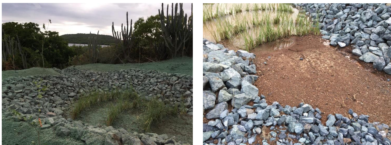
Figure 41. Example of a sediment trap built by PDC in Culebra Puerto Rico.
