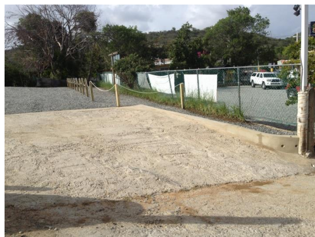
Figure 32. Gravel filter and parking lot stabilization by PDC in Parguera, Puerto Rico.
