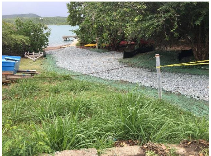
Figure 26. BMP's implemented following a train treatment approach in Fulladosa Culebra, Puerto Rico. Practices include bioswales and raingardens.
