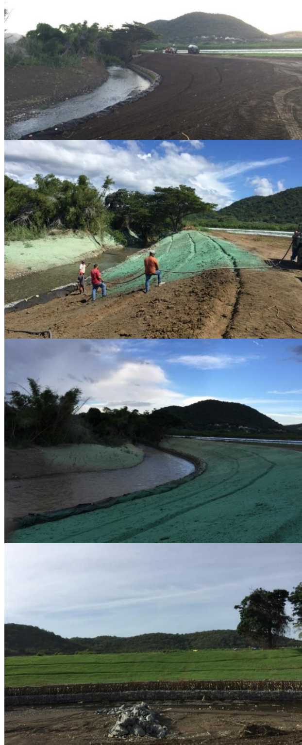
Figure 38. Hydroseeding implementation by PDC on a riverbank stabilization project in the Río Loco, Guánica Puerto Rico
