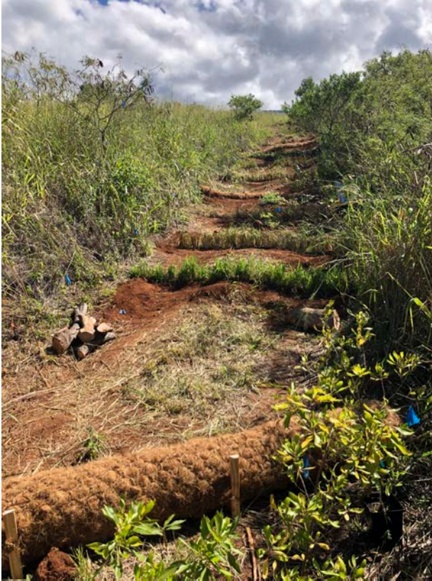
Figure 2 BMP treatment train
