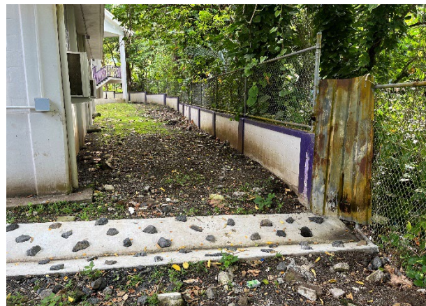
Paved flume drains to stream. Adjacent green space could be used for storage and treatment of stormwater runoff.
