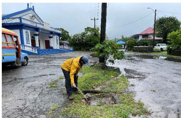
Water ponding in front of Catholic Church and turbid water entering catch basin
