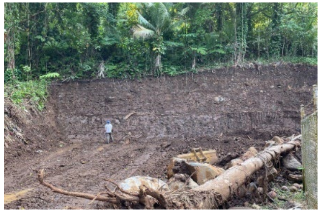
Cut slope close to edge of Rt. 006 behind water tank and other erodible soils at site should be stabilized (Site #6).
