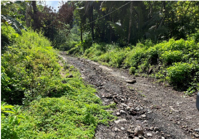
Rutting of unpaved access road/driveway (Site #7) is Erosion gully along unpaved driveway. This could be fixed with regrading of surface to an insloped pitch and installation of a ditch.
