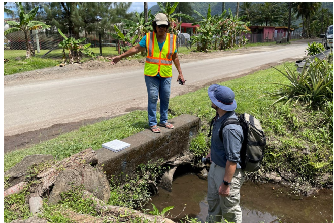
Culvert near Origin Gas that may be undersized.
