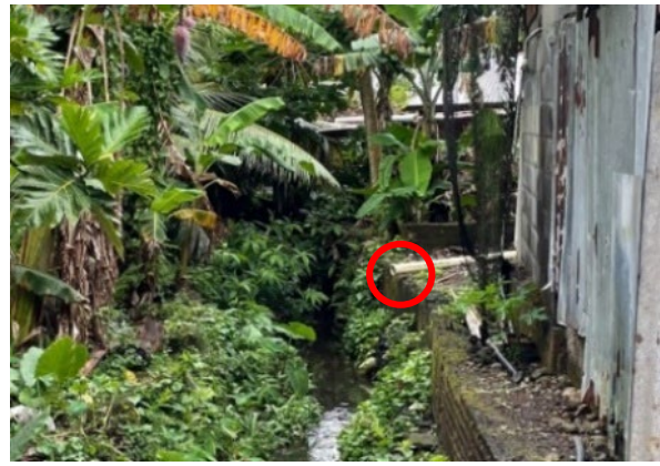
Identify remaining discharges piped directly to stream. If this is laundry or sink/shower wash water, then it should be targeted for hook up to the new sewer line.
