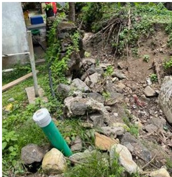
New sewer line cleanout installed at a home in Aua.
