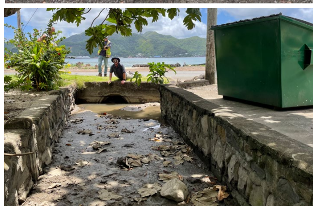
Two clogged drain inlets on Route 006 are causing long-term ponding on the road (I-64, top), erosion, and sediment contributions to road inlets downhill (I-51, middle). A blocked culvert pipe at I-16 causes backup in the stream and contributes to flooding at PT-Mart and Laundry (bottom).
