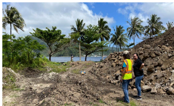
Stockpiled stone with in adequate erosion controls near shoreline at Onesosopo Park
