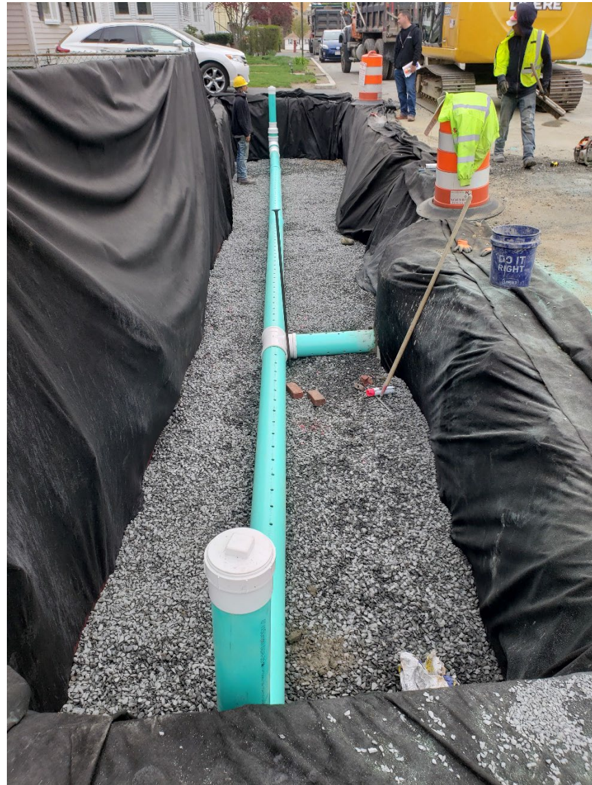
Tree Trench Gravel Reservoir During Construction – Watetown, MA
