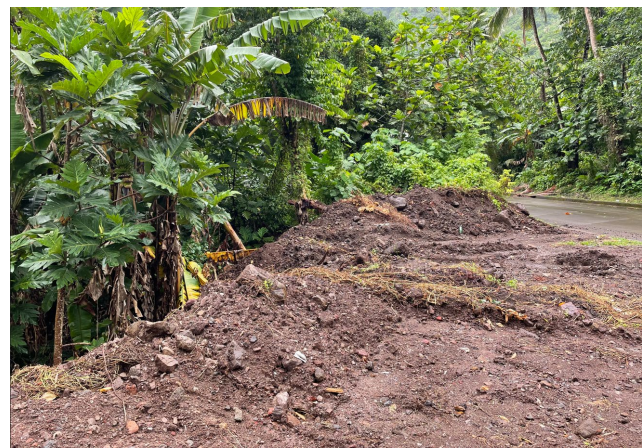
(LEFT) Automobile shop and lot. (RIGHT) Excavated material cast downslope at Water Tank construction site.
