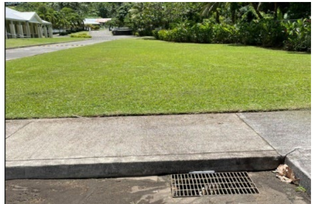
Convert existing lawn area to vegetated filters that can clean parking lot runoff before discharging into existing storm drain at the Mormon Church Site #9.
