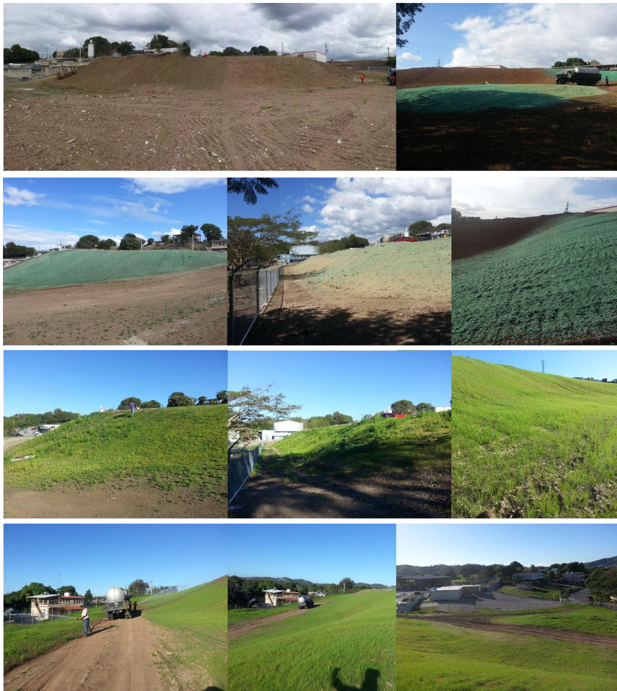
Figure 18. Hydroseeding process on one of the multiple Hydroseeding sites of the GB/RL Watershed.
