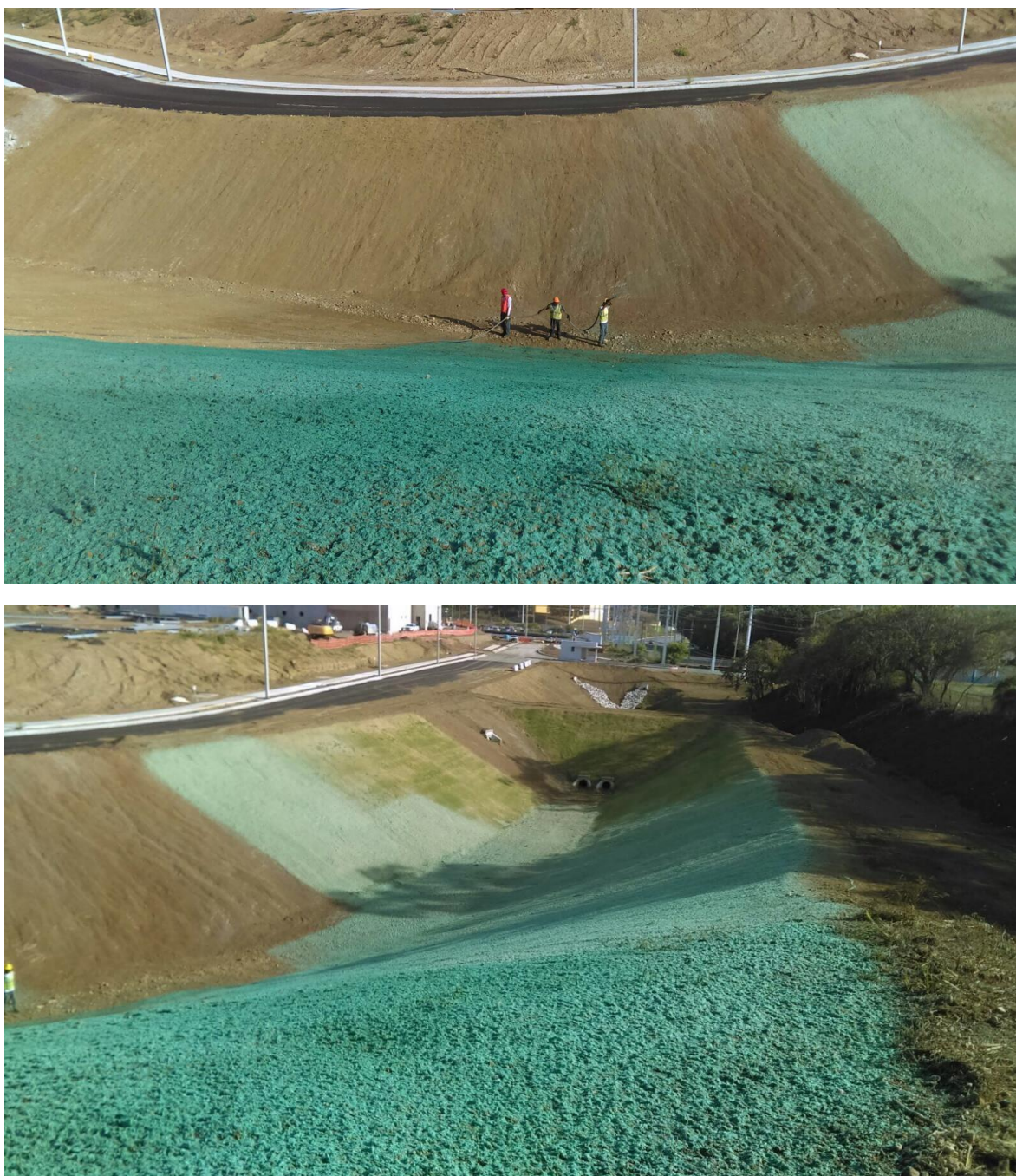
Figure 56. Images during Hydroseeding implementation of Sartorius Plant Expansion Project in Yauco Puerto Rico.
