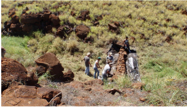
Figure 4.2: Sediment dam underway.
