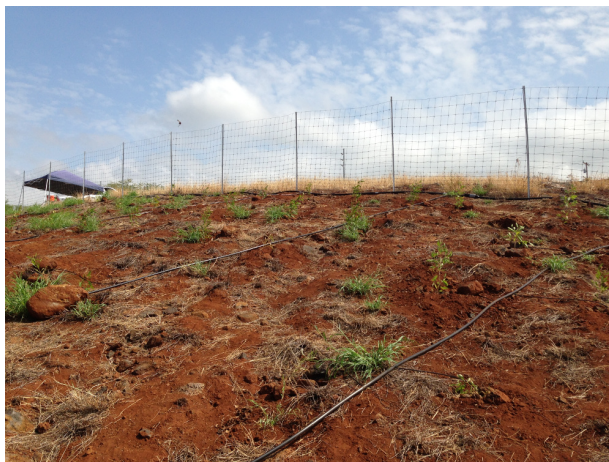
Figure 6.1: New fence, irrigation lines, and plants..
