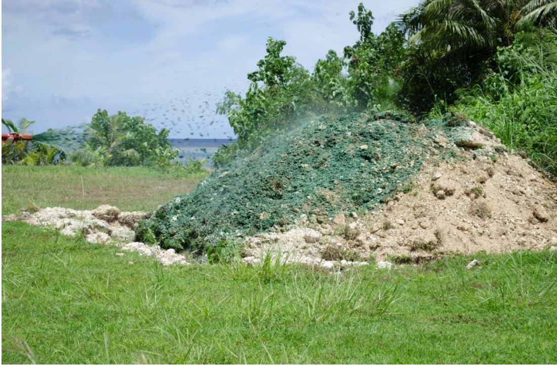
Figure 46: Hydroseeding
