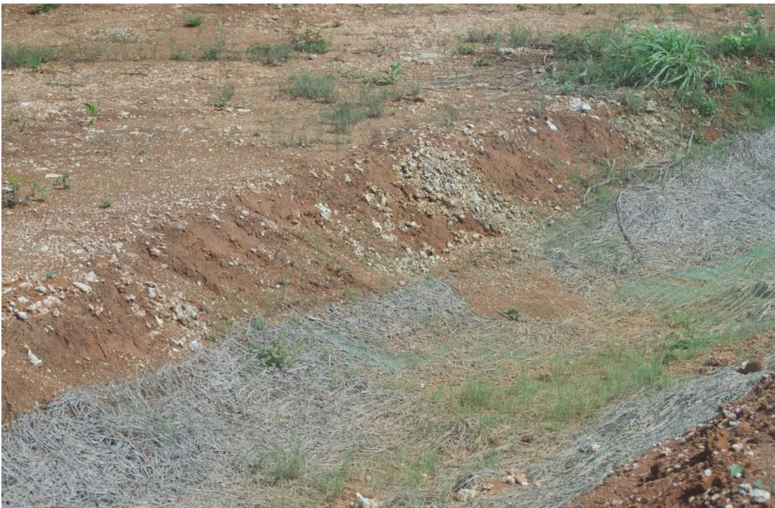
Figure 47: Erosion Control Blankets
