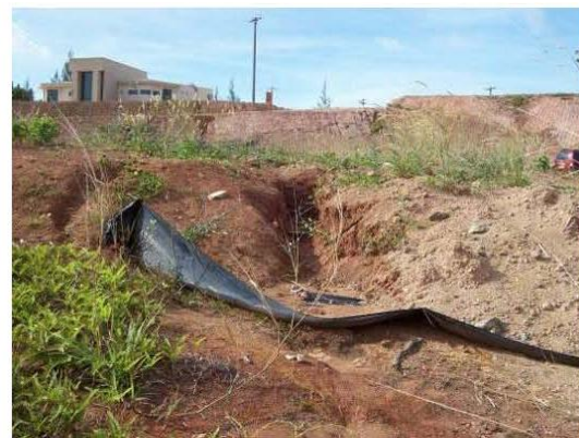
Figure 38. Exposed soil (left) and deep gullies (right) on a development site on J Street on Nimitz Hill in 2008. Silt fences were not effective as they did not trap the eroded sediments from the gullies and nearby areas. Photos courtesy of CWP/HW (2010).
