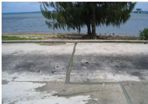
Figure D-12. Runoff from the concrete bus loop is conveyed across the concrete pad via grooves and sheetflow, and discharges through square notches in the curb to the nearby beach and water. There are oil stains on the concrete pad and bus exhaust deposits other pollutants on the concrete.
