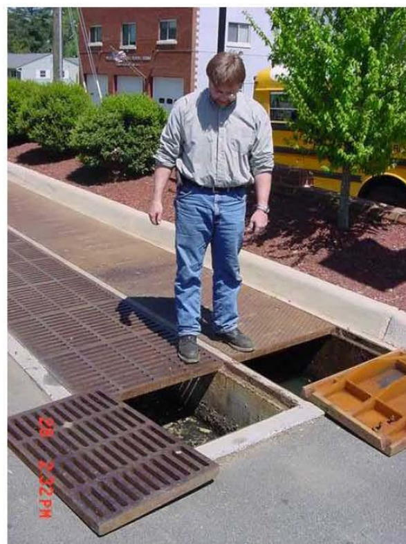
Figure D-15. Example of sand filter with grate top. The grates provide maintenance access.
