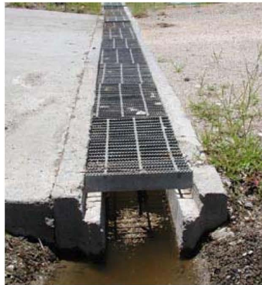
Figure D-24. Example of a trench drain that can be used to convey runoff from parking area to bioswale.
