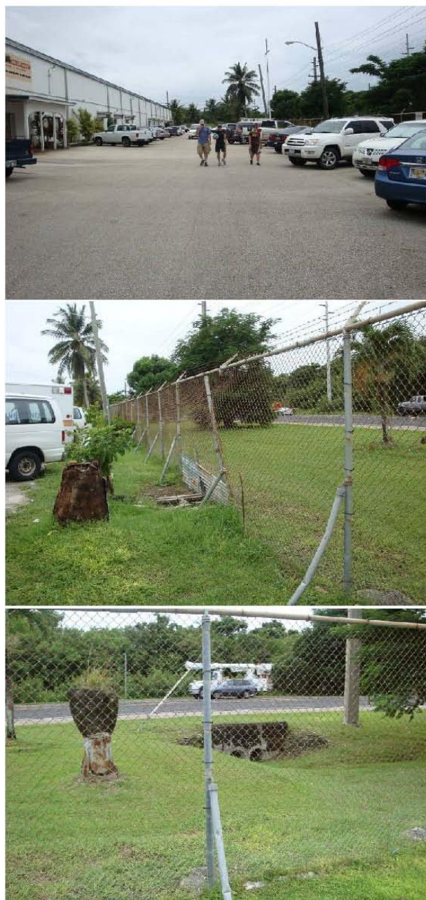
Figure D-1. Runoff from portion of rooftop and front parking drain to grassed area, then through culvert under Marine Corps Dr.
