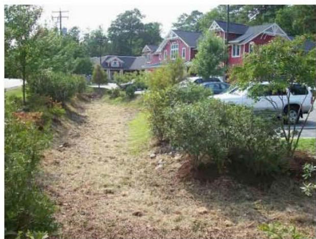
Figure D-14. Example of a surface sand filter treating parking lot runoff.
