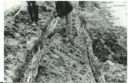
Live Fascine Installation
