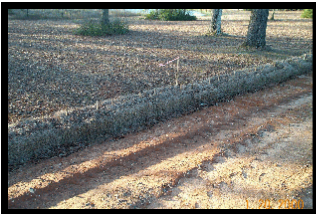
Exhibit 6.1a - Improper use and/or installation of hay bale dikes.
