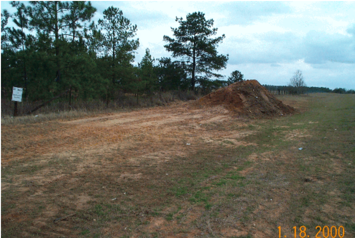
Soil stockpile located on the crest of a hill where runoff is minimal
