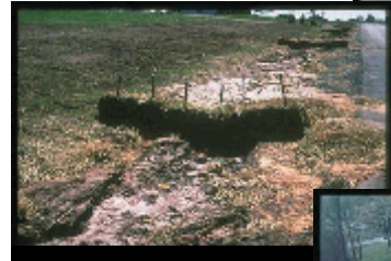
Improper Construction, Ineffective Installation, and Mis-application (Concentrated Flow)
