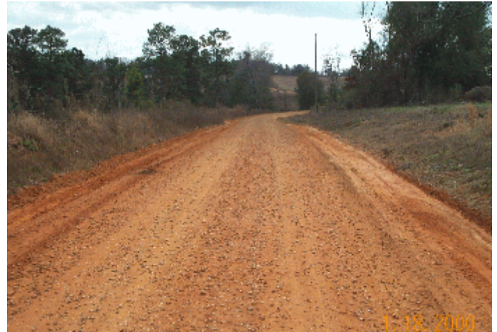
Exhibit 1.1b - Examples of 0" to 1/4" crown with no road ditches in place. Water infiltrates the soil of the sandy and flat road surface minimizing runoff from the roadway. The water that sheds from the roadway is readily removed from the road surface into the roadway edges allowing a passable lane in the center of the roadway.
