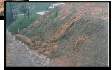
Exhibit 6.1a - Improper use and/or installation of hay bale dikes.
