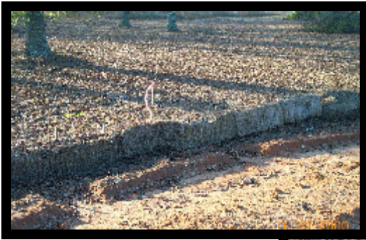
Poorly Installed Hay Bales
