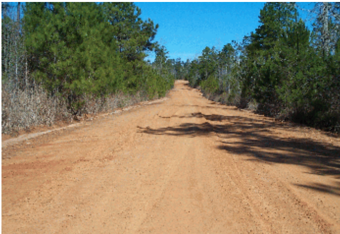
Unnecessary Blading. Road is adequate.
