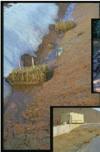
Poorly Installed Hay Bales
