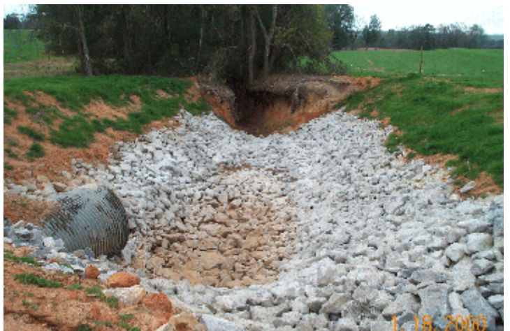
Exhibit 4.1b - Depressed-type plunge basin at culvert discharge with transition apron to outlet channel.
