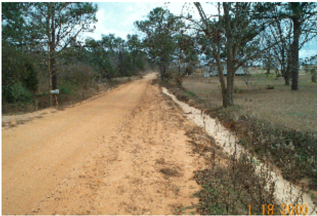
Flat Bottom (Trapezoidal) Shaped Ditch
