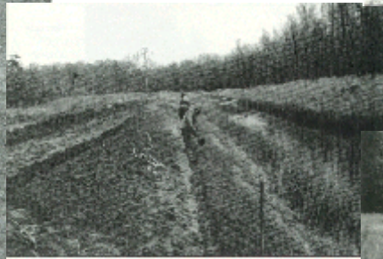
Bank Trenching for Fascine Installation
