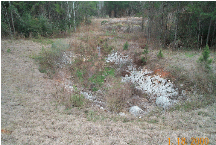
Exhibit 4.1b - Depressed-type plunge basin at culvert discharge with transition apron to outlet channel.
