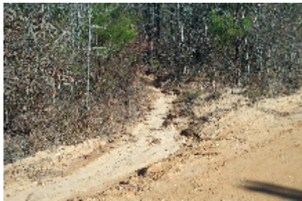
Turn-out to a drop inlet.
