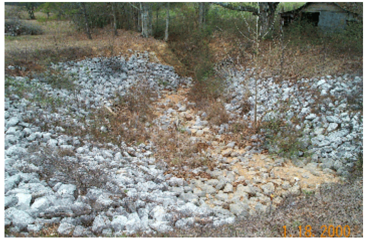
Exhibit 4.1a - Depressed-type energy dissipating basin at culvert discharge with transition apron to outlet channel.
