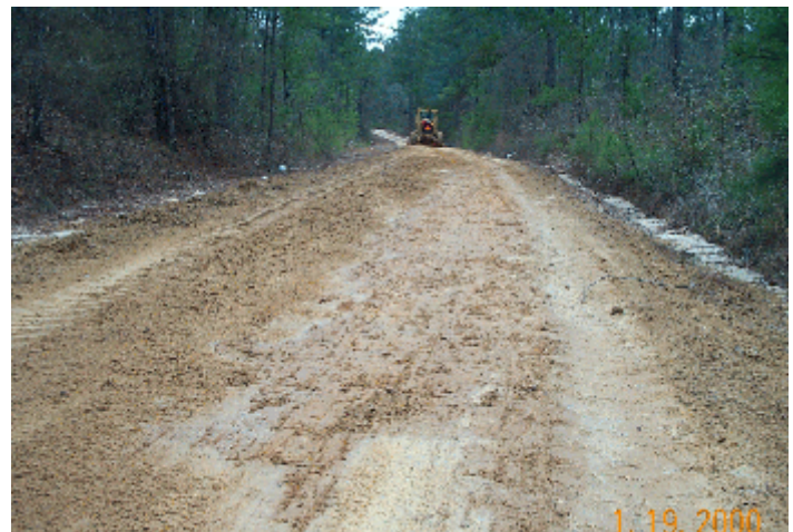
Unnecessary Blading. Road is adequate.
