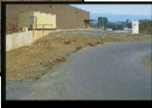
Exhibit 6.1a - Improper use and/or installation of hay bale dikes.
