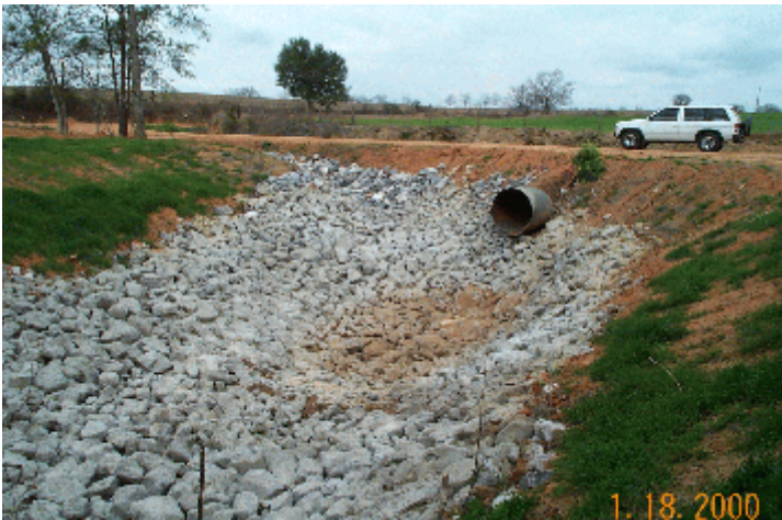
Exhibit 4.1b - Depressed-type plunge basin at culvert discharge with transition apron to outlet channel.
