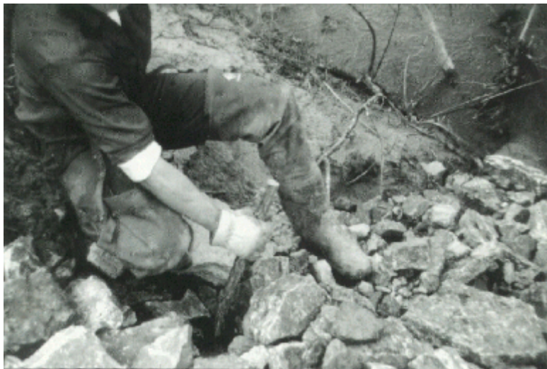
Vegetated Riprap Revetment by Design
