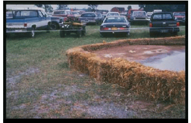
Exhibit 6.1a - Improper use and/or installation of hay bale dikes.
