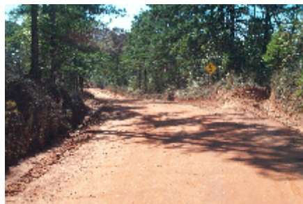
Turn-out at gradient changes.
