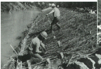
Brush Mattress Installation
