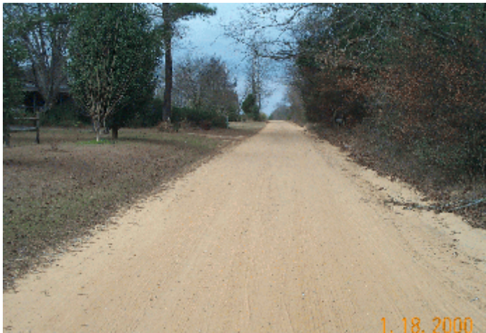
Exhibit 1.1b - Examples of 0" to 1/4" crown with no road ditches in place. Water infiltrates the soil of the sandy and flat road surface minimizing runoff from the roadway. The water that sheds from the roadway is readily removed from the road surface into the roadway edges allowing a passable lane in the center of the roadway.
