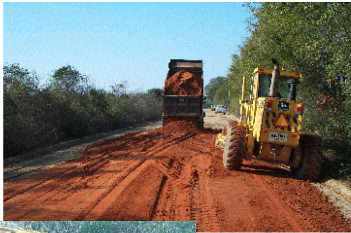
Clay blended into roadway surface with scarifier and blade
