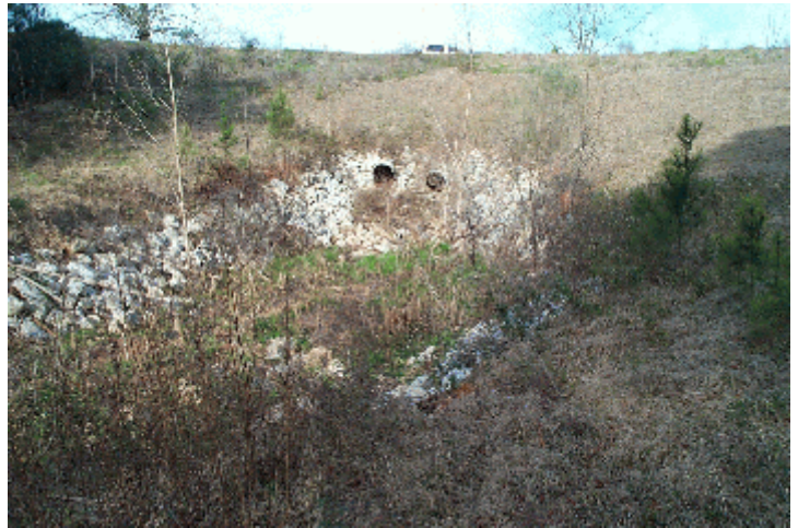
Exhibit 4.1b - Depressed-type plunge basin at culvert discharge with transition apron to outlet channel.
