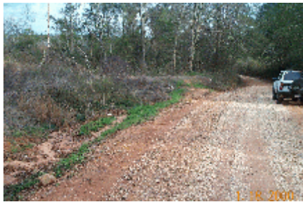
Turn-out to a drop inlet.
