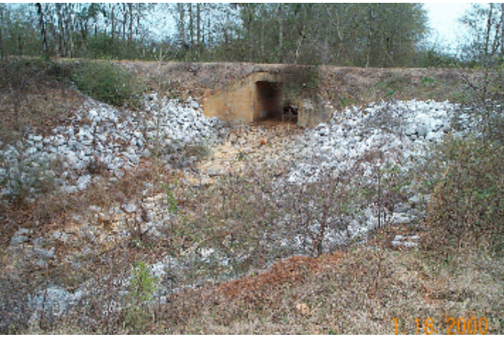
Exhibit 4.1a - Depressed-type energy dissipating basin at culvert discharge with transition apron to outlet channel.
