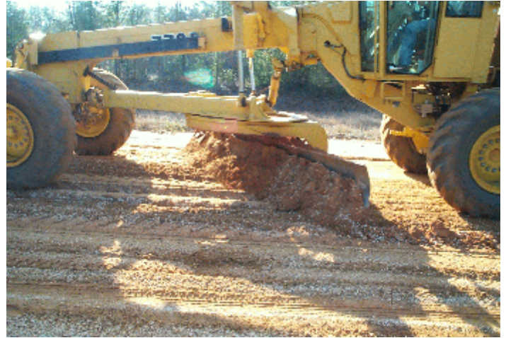
Proper blade angle and wheel lean.
