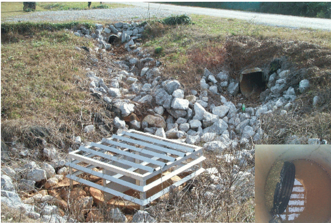
Exhibit 4.2 - Drop Inlet/Box/Manhole
