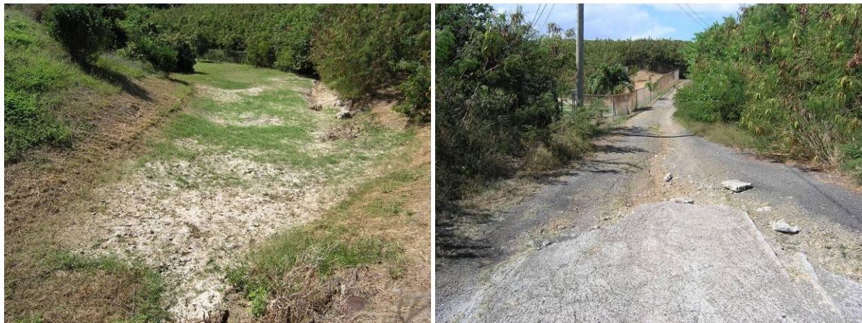
Figure 4.29. A pond is located upstream from the culverts – dry at the time of observation (left). The road itself is deteriorating and providing a sediment load to the gut (right).
