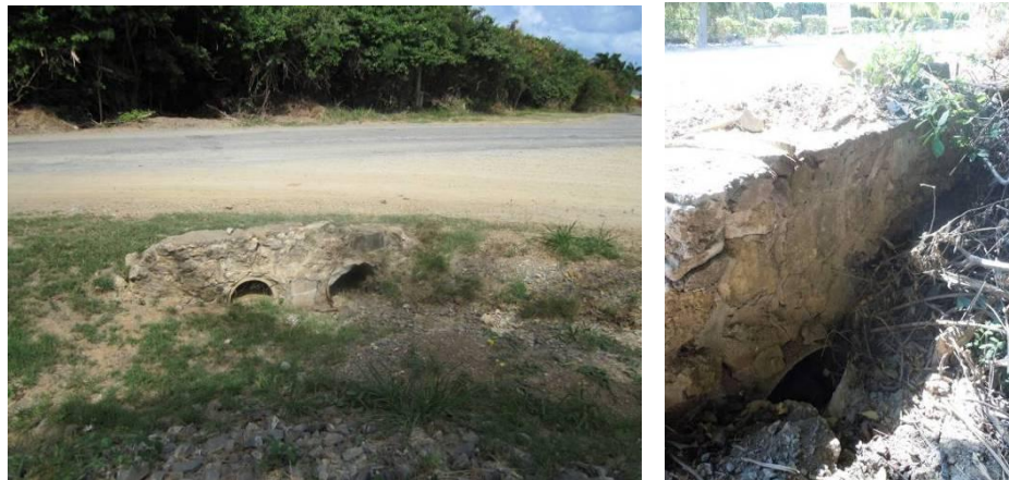
Figure 4.6. The two culverts that carry flow from Seven Flags Rd. and a portion of East End Rd. to Solitude Bay blocked with sediment on both the upstream (left) and downstream ends (right).
