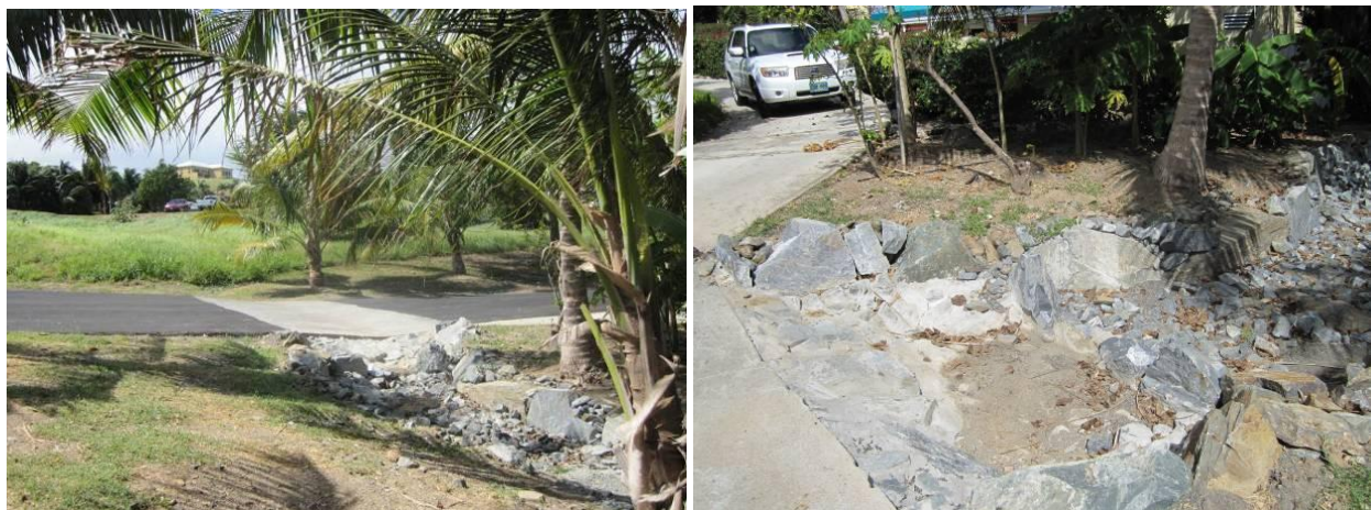
Figure 4.21. Stormwater flows from the grass depression and the cul-de-sac to a riprap-lined channel (left). A sediment forebay was constructed with a rock weir (right).
