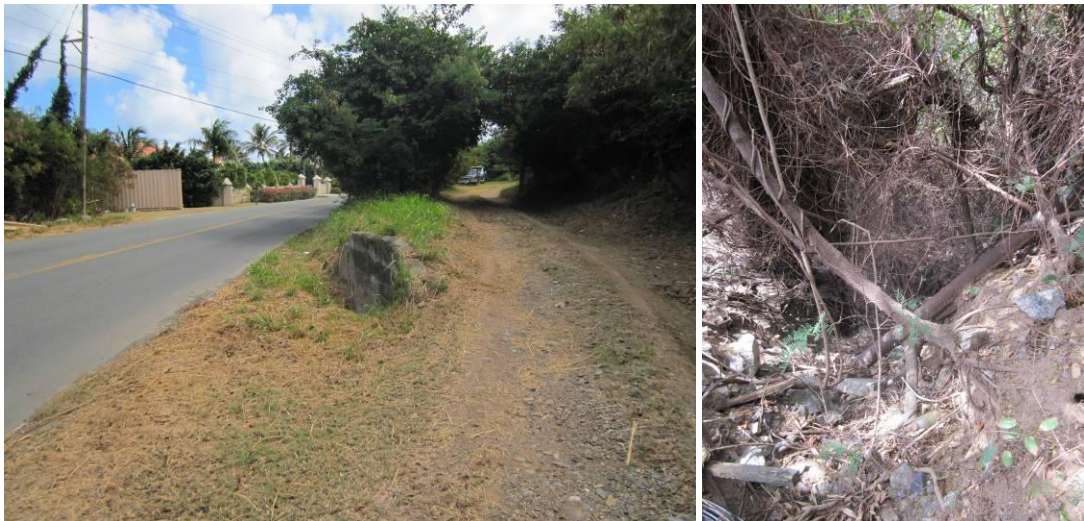
Figure 4.34. Upstream end of culvert has large headwall separating it from an unpaved drive (left); the downstream end is scoured out and clogged with vegetation (right).
