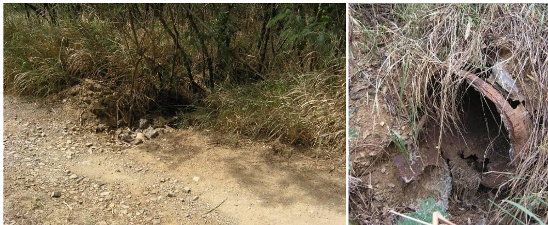
Figure 4.26. The upstream end of this ductile iron culvert is completely blocked (left). The downstream end is corroded and disintegrating (right).
