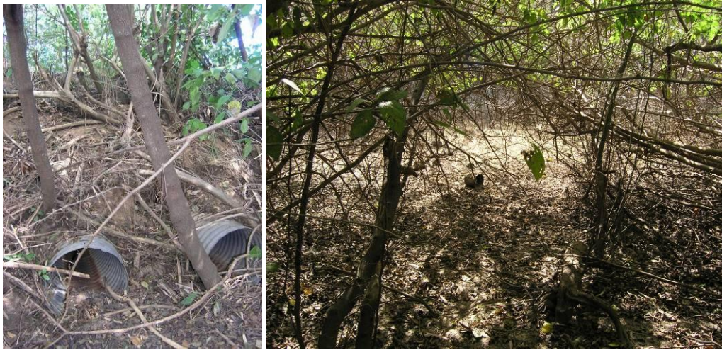
Figure 4.24. Two 24-inch CMP culverts that cross an unnamed road (left). A depression exists at the upstream end that only holds water in the wet season (right).
