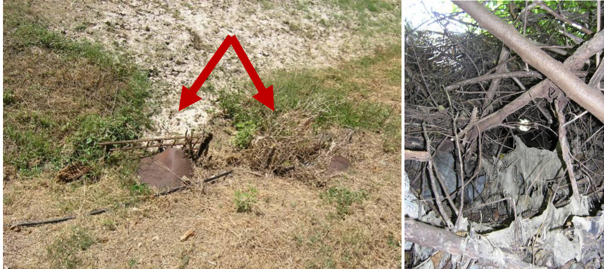
Figure 4.28. The two 24-inch ductile iron culverts have damaged trash racks – one made of rebar grate and one made of wire fencing and sticks (left). The downstream end is clogged with vegetation (right).
