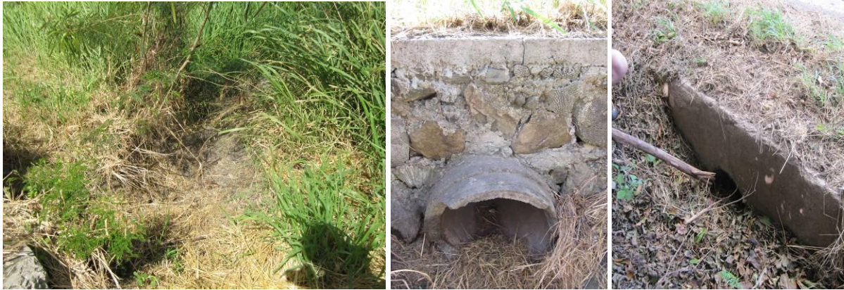
Figure 4.33. Erosion downstream from the first culvert (left); the second, chipped culvert (middle); and the partially blocked third culvert (right).
