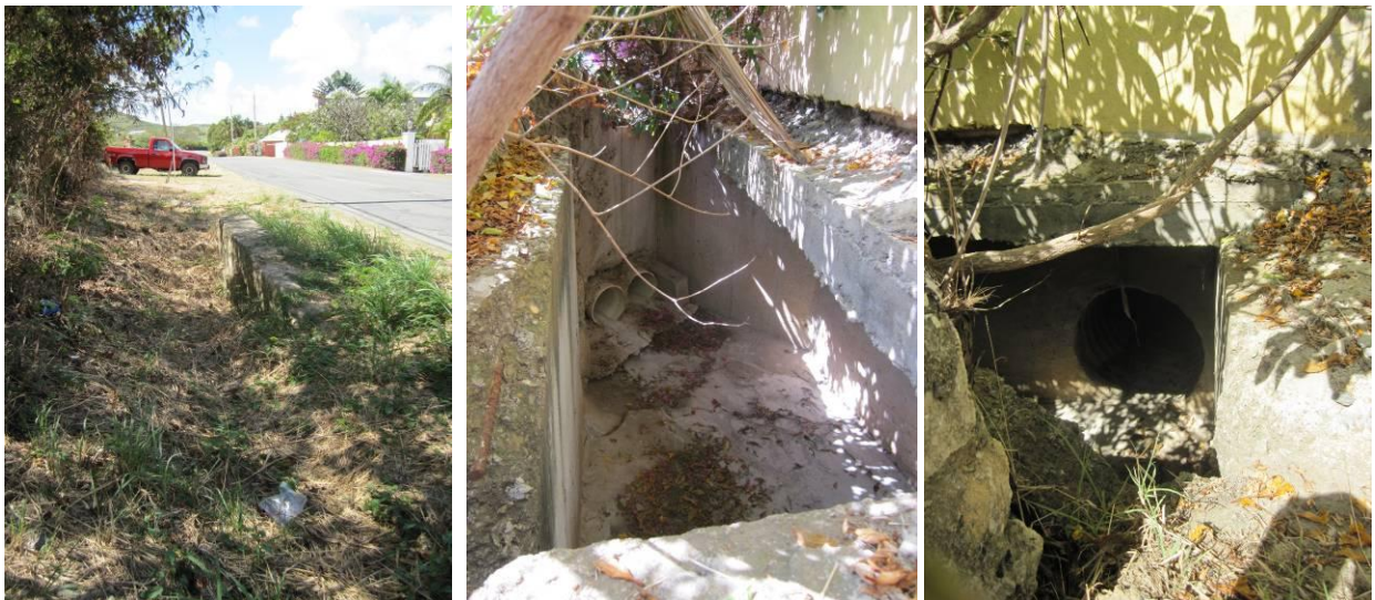
Figure 4.36. Upstream end of 24-inch culvert and headwall; Sierra Verde Rd. in the background (left); the two PVC pipes in the drainage structure at the downstream end of the culvert (middle); and the ultimate discharge pipe to the bay where runoff leaves the drainage structure (right).
