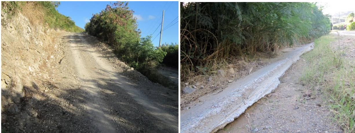
Figure 4.4. Roads in the Hope and Carton Neighborhood are unpaved and very steep (left). Runoff from this road bypasses and undermines the paved swale (right).
