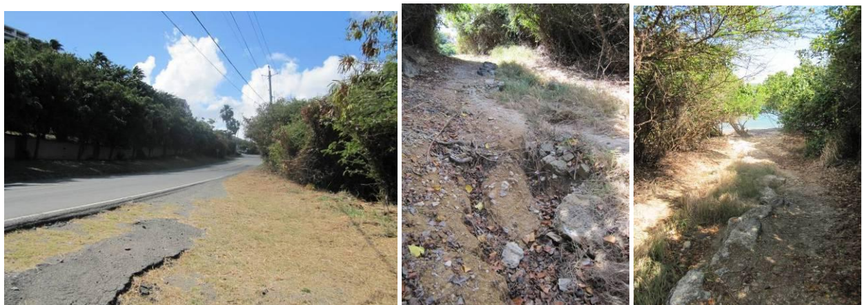
Figure 4.19. Runoff from Coakley Bay Condos flows across East End Rd. and down a beach access road (left) causing erosion gullies (middle), and this sediment-laden runoff enters Coakley Bay (right).
