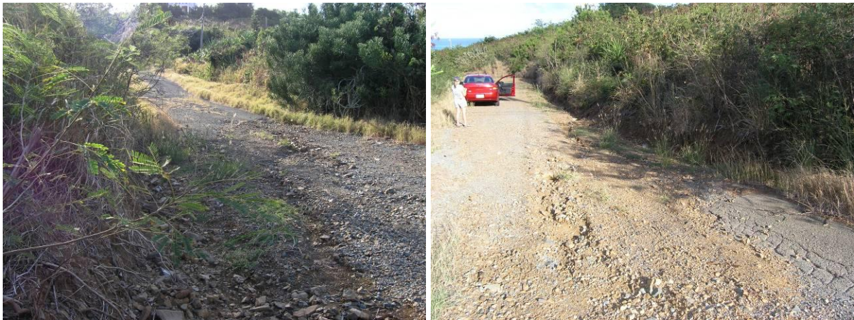
Figure 4.3. Erosion gully at the transition from paved driveway to unpaved private road looking up-gradient (left) and down-gradient (right).
