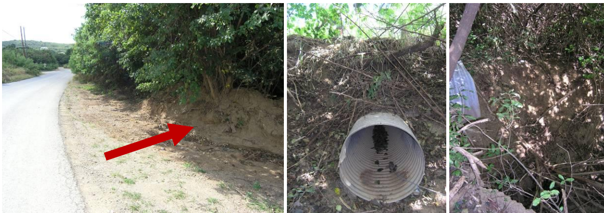
Figure 4.25. The arrow shows the sediment that gets cleared off Pony Club Trail and pushed into the gut (left). The upstream end of the culvert is clear of debris and is in generally good shape (middle); however, a large scour hole has formed at the downstream end (right).
