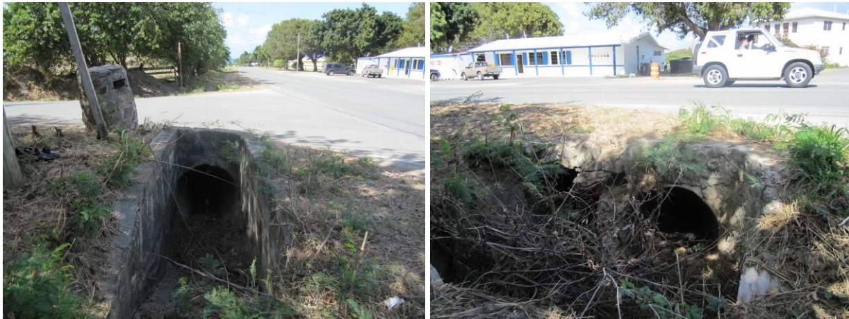
Figure 4.14. 30-inch culvert under Solitude Rd (left) and two 30-inch culverts under East End Rd., leading to a 48-inch culvert that discharges to Coakley Bay (right).
