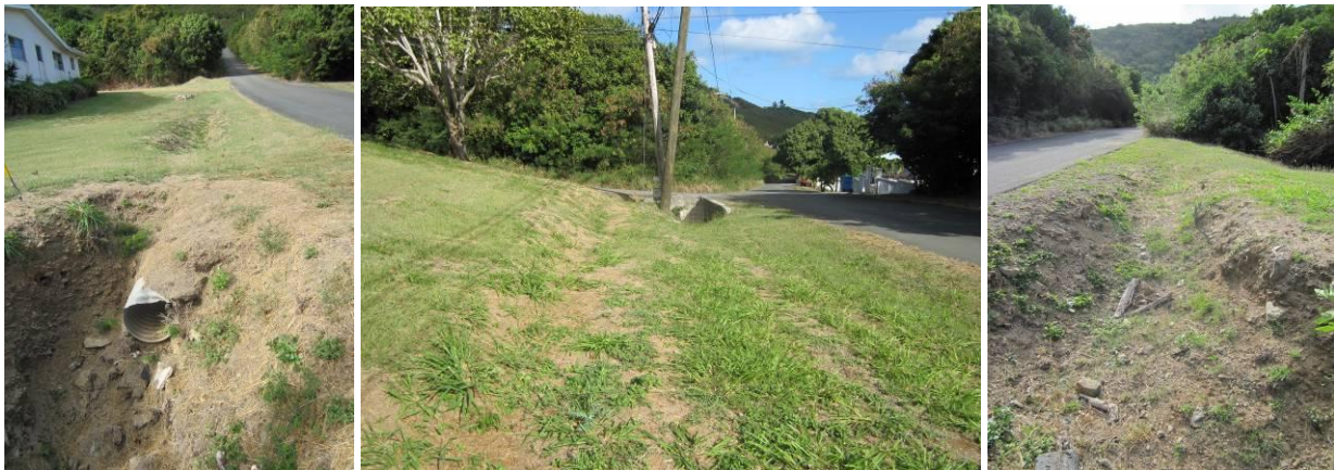
Figure 4.32. Erosion caused by deteriorating culverts in the southern portion of Pleasant Valley.
