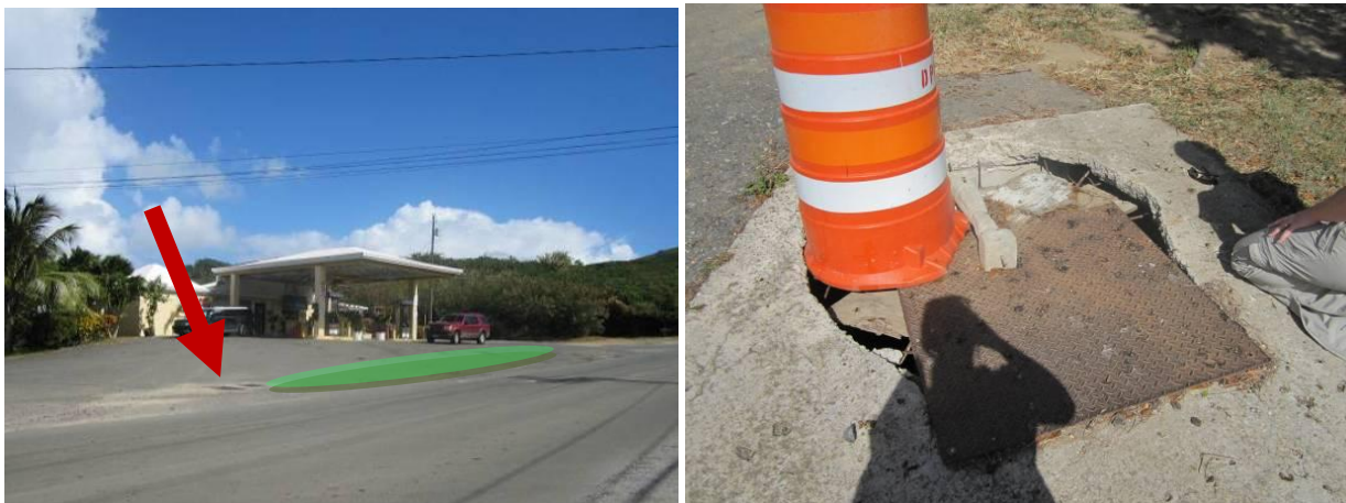
Figure 4.15. Some pavement could be removed at the gas station to create a treatment swale (shown in green) up-gradient from the existing catch basin indicated with an arrow (left). Manhole covers are missing all along the 48-inch culvert leading out to Coakley Bay, creating a safety hazard (right).
