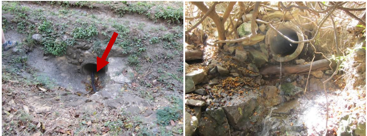
Figure 4.18. Arrow indicates PVC pipe discharging dry weather flow into culvert (left). Dry weather flow observed at downstream end (right).
