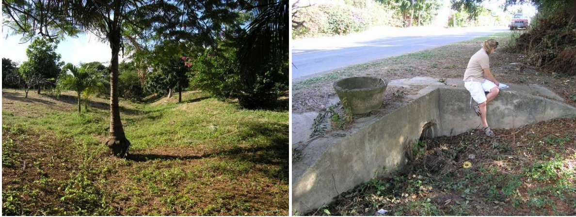
Figure 4.12. View upstream along one fork of the gut system (left). Concrete headwall for 15-inch reinforced concrete culvert (right).
