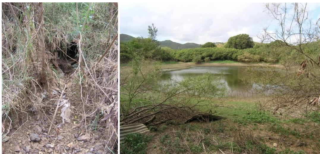
Figure 4.27. Scouring was observed downstream of this culvert (left), which leads to sedimentation of the large pond downstream (right).
