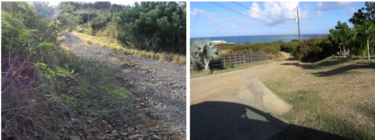
Figure 4.37. Erosion along private road within Sierra Verde neighborhood at meeting point between paved and gravel roadways (left) and water bar installed along main dirt road in Sierra Verde neighborhood.
