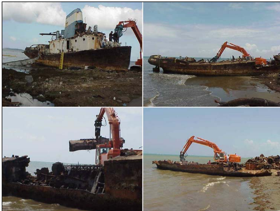
Figure 2. The M/V Kimton being dismantled in place.
