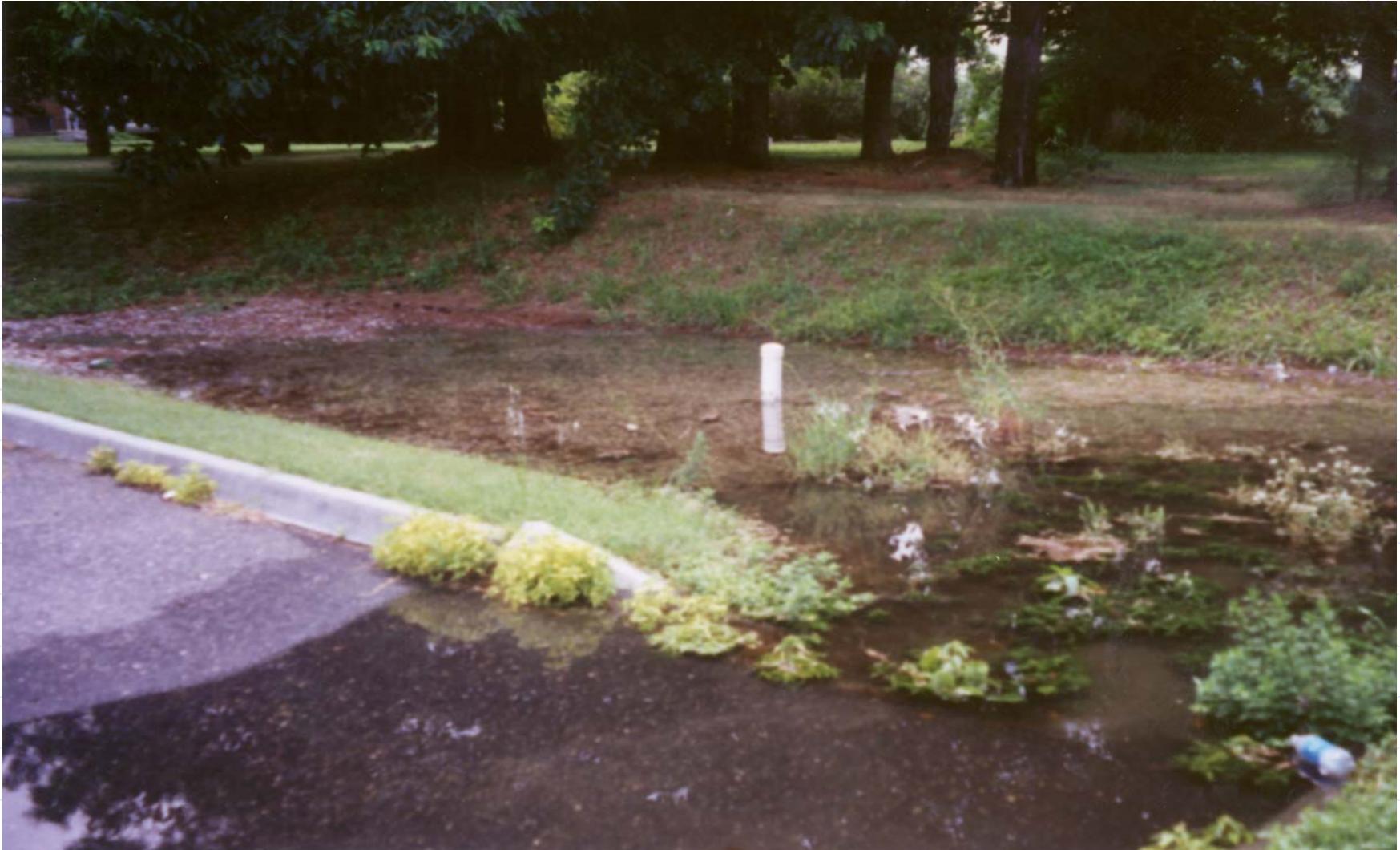
Nominee No. 2: The infiltration trench that couldn't
