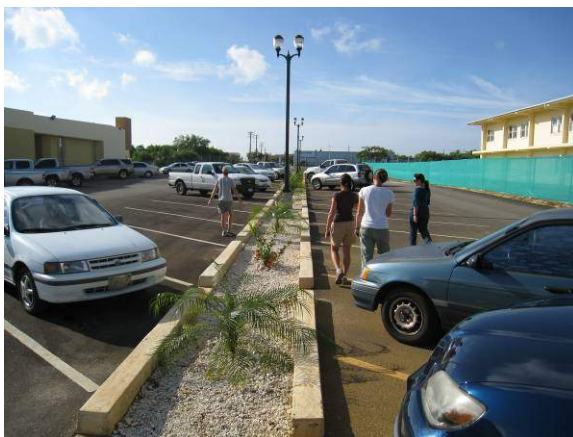
Figure S2.2. Coral stone filter in a parking lot (Note: designs built according to this specification would likely be wider and incorporate additional materials)
