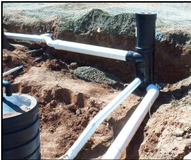
Figure S4.7. Installation of Vortex Filter prior to backfill
