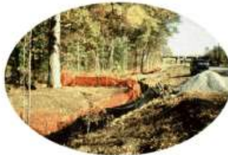
5. Erosion & Sediment Control
