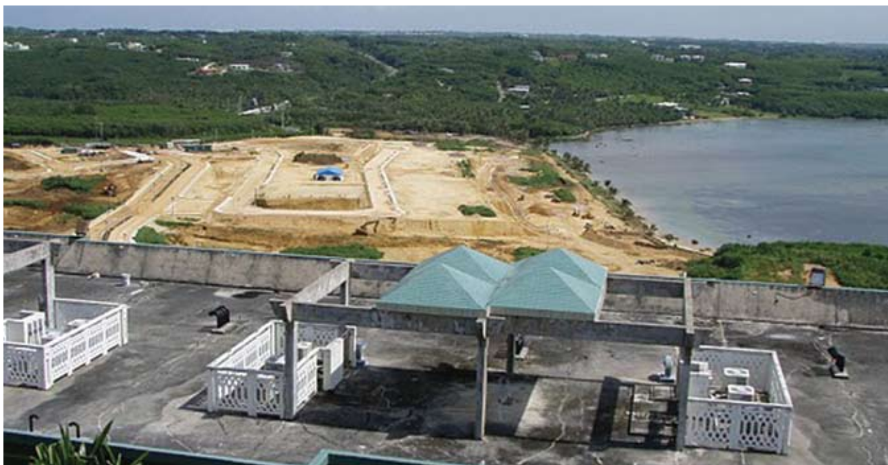
Development activities are increasing in anticipation of the military build-up in Guam. It is important that proper mitigation planning is set in place when impacts to coral ecosystems can not be avoided. Photo Credit: Kathy Chaston, NOAA CRCP
