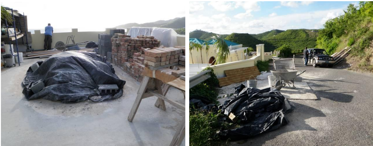
Figure 12. Effective and non-effective material management on small construction sites
