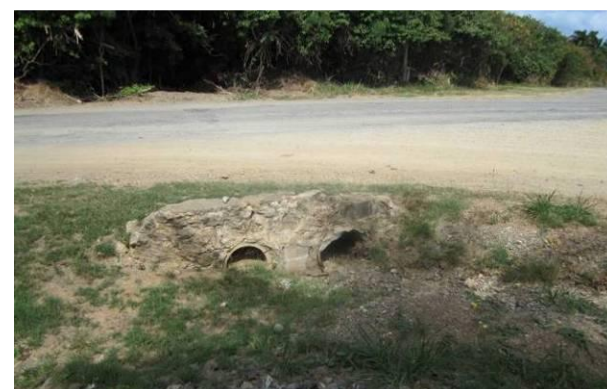
Existing culverts under East End Rd.
