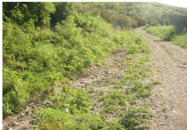
Space alongside road to install stepped/check dam system.
