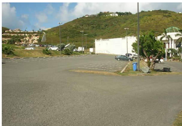
Parking lot landscape island for proposed conversion to rain garden, which would provide additional pretreatment for detention basin.
