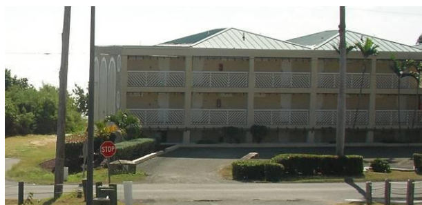
Small parking lot and landscaped area proposed for permeable pavement and rain garden.
