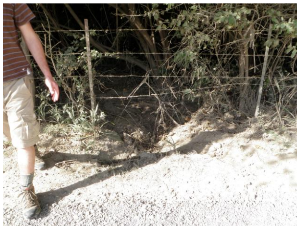
Sediment deposition at outlet location.
