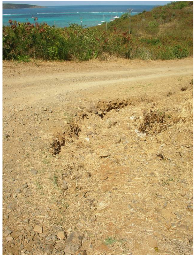
Erosion along ditch at bend in road.
