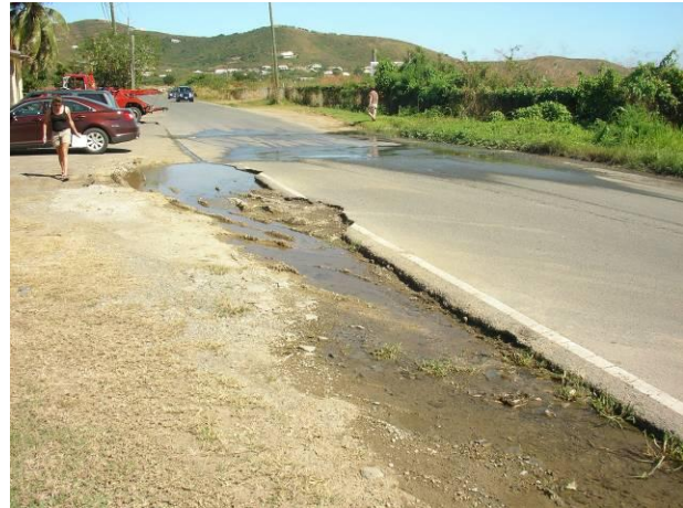
Location at Milgie's where East Gut flow is diverted along the parking area and then across Rt. 624 via an existing paved dip.
