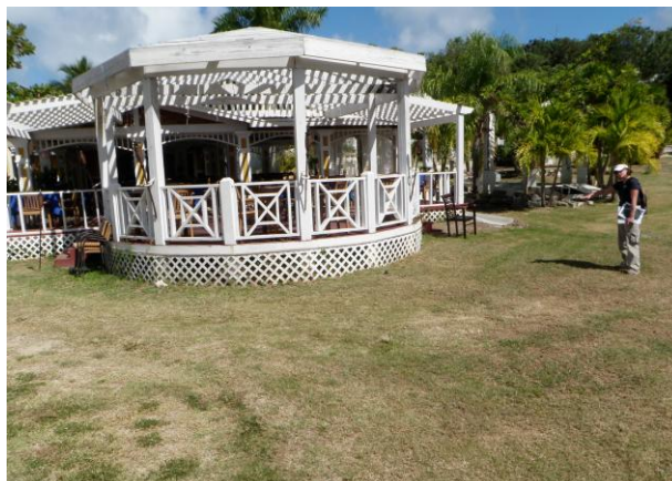
Proposed area for rain garden installation. Extend existing paved flume and install gutter and downspouts to convey flows to sediment forebay.
