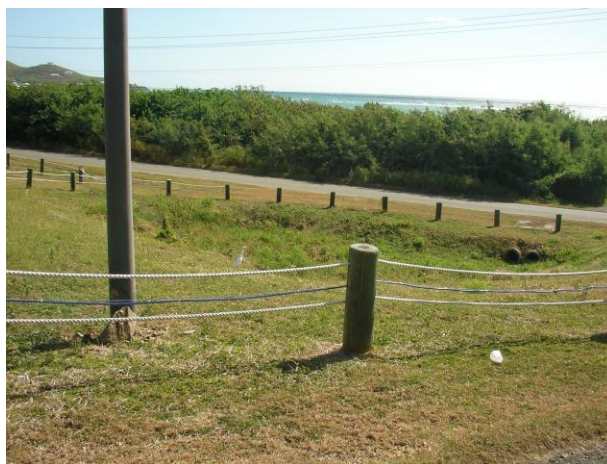
Existing detention basin with double outlet pipes along South Shore Rd.
