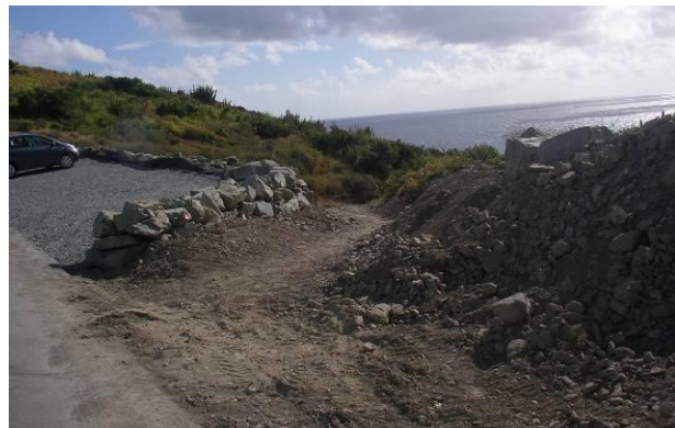
Newly installed parking lot and trailhead.
