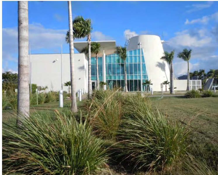
Figure 6. UVI RTPark 64 West Center provided a great opportunity to demonstrate green building features. .
