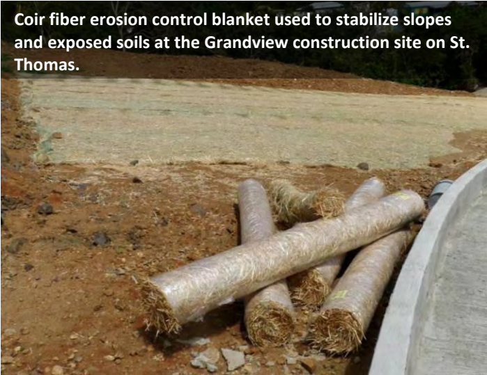
Figure 8. Example of materials that can be used to stabilize slopes.
