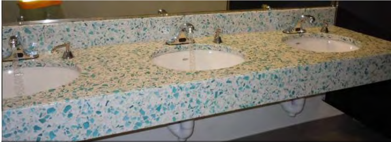
The recycled glass used for sink counter tops in bathrooms as well as recycled cardboard stall partitions illustrate some of the material reuse principals of green design.
