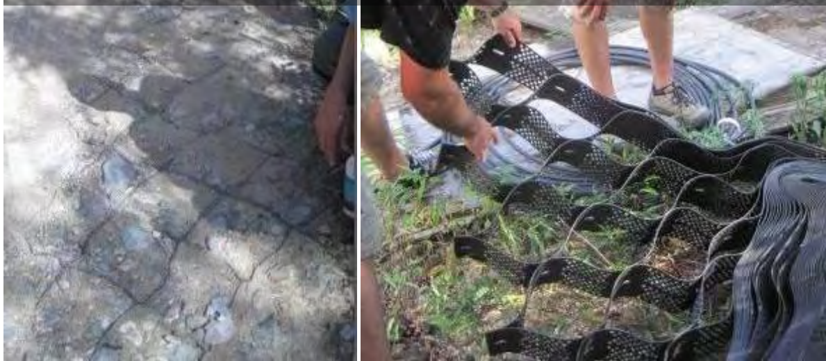
Photos of Geoweb installation at UVI campus on St. Thomas.
