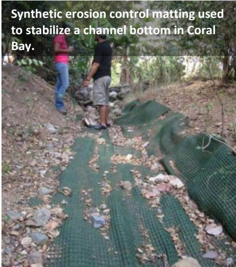
Figure 8. Example of materials that can be used to stabilize slopes.
