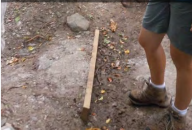
Diversion berm installed on beach access trail to direct stormwater into vegetated swale/basin rather than direct discharge to the beach.
