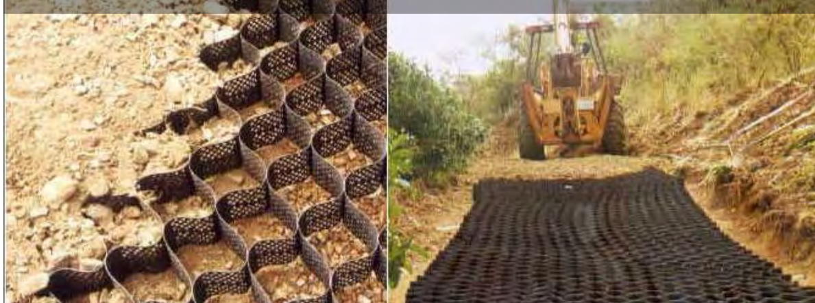
Photos of Geoweb installation at UVI campus on St. Thomas.
