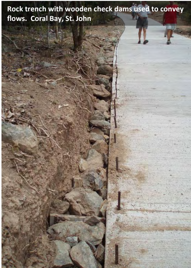
Figure 6. Examples of road-side conveyance systems.
