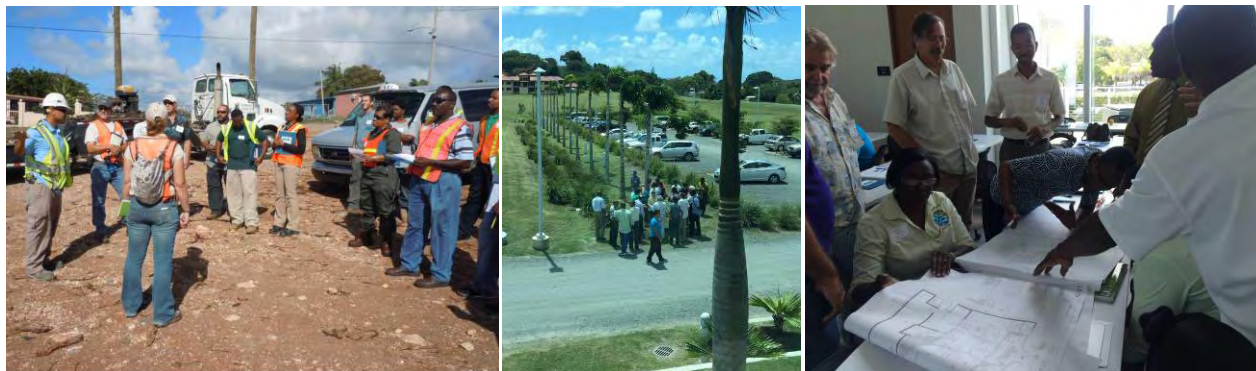
Participants in the two workshops visited construction sites, toured a LEED-certified building, and participated in classroom activities.
