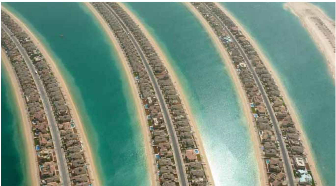
The Gulf's densely populated, and predominantly sandy, easily erodible, and low-lying coastal regions are especially vulnerable to the impacts of sea level rise through direct inundation, erosion and salt water intrusion. Infrastructures on offshore developments, such as these villas on the fronds of Palm Jumeirah, are also at risk. Credit: Imre Solt, Dubai Constructions Update ( www.imresolt.com )
