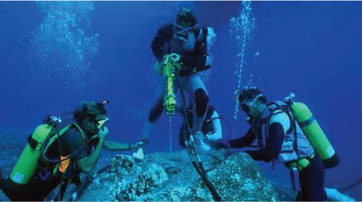
Divers prepare substrate for placement of mooring bouys.
