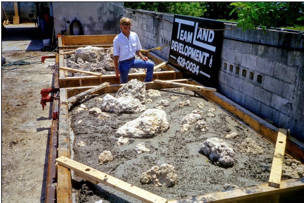
Figure 5. Pre-cast concrete and limestone boulder armor unit used in the Maitland restoration (photo credit: Harold Hudson NMSP/NOAA).
