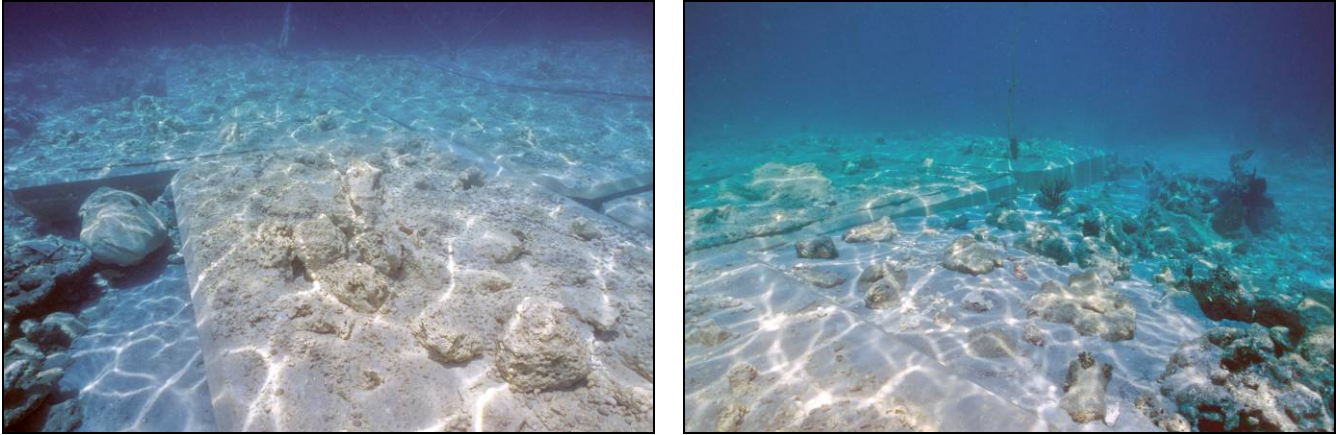
Figure 7. Completed restoration with armor units (left) and “puddle pour” with limestone “dressing” stones (right) (photo credits: Harold Hudson NMSP/NOAA).
