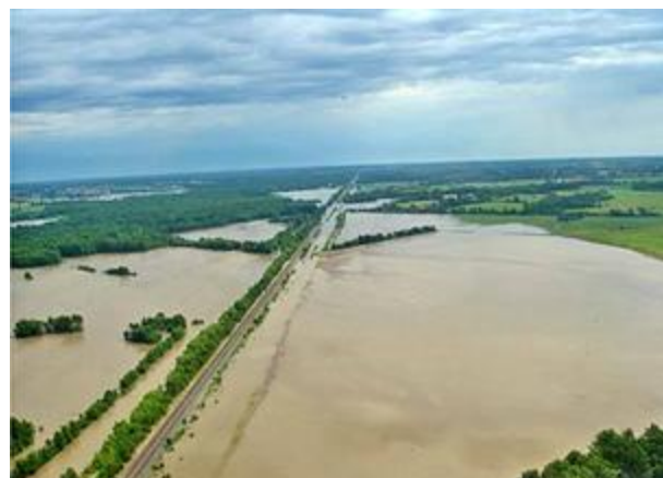
Aerial view of flooded railway
