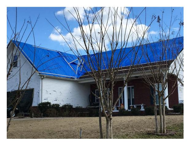
**Image 2.** Common damage to roof and siding observed at the Fox Meadows Subdivision on the southeast side of Cullman, Alabama.
