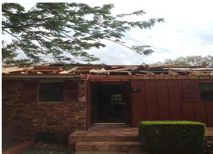
A home in Plaska had its roof removed by intense straight-line winds associated with a supercell. Photo courtesy KFDA news.
