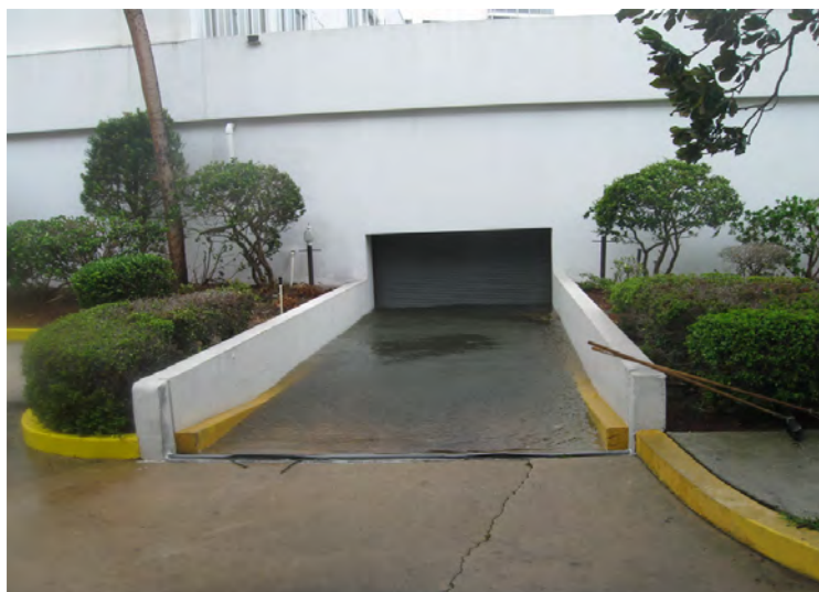
A parking garage at 1596 Lancaster Terrace in Jacksonville was flooded.
