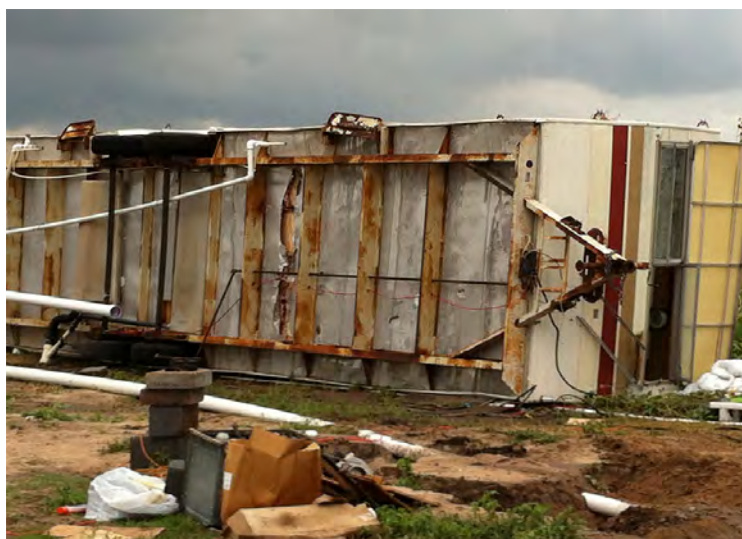
Rolled, unanchored trailer home at a colonia (makeshift neighborhood of migrant workers along the U.S./Mexico border) after an estimated 60 to 65 mph microburst passed through, near Doolittle, TX.
