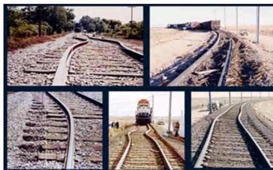
**Figure 7:** Railway Buckling
