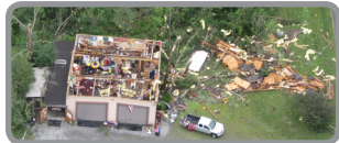
Above: EF-2 tornado damage in Erie County, NY, on July 20. Credit: NWS BUF.
